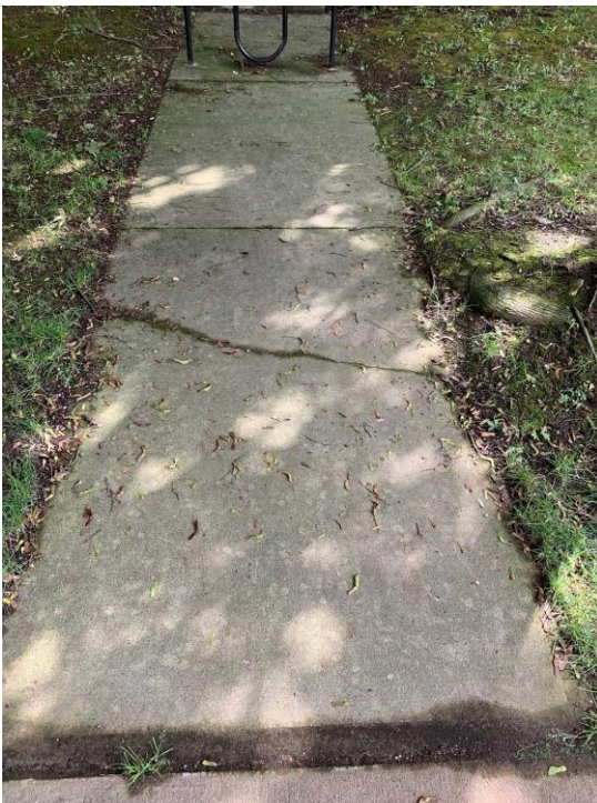
West Side of Building
