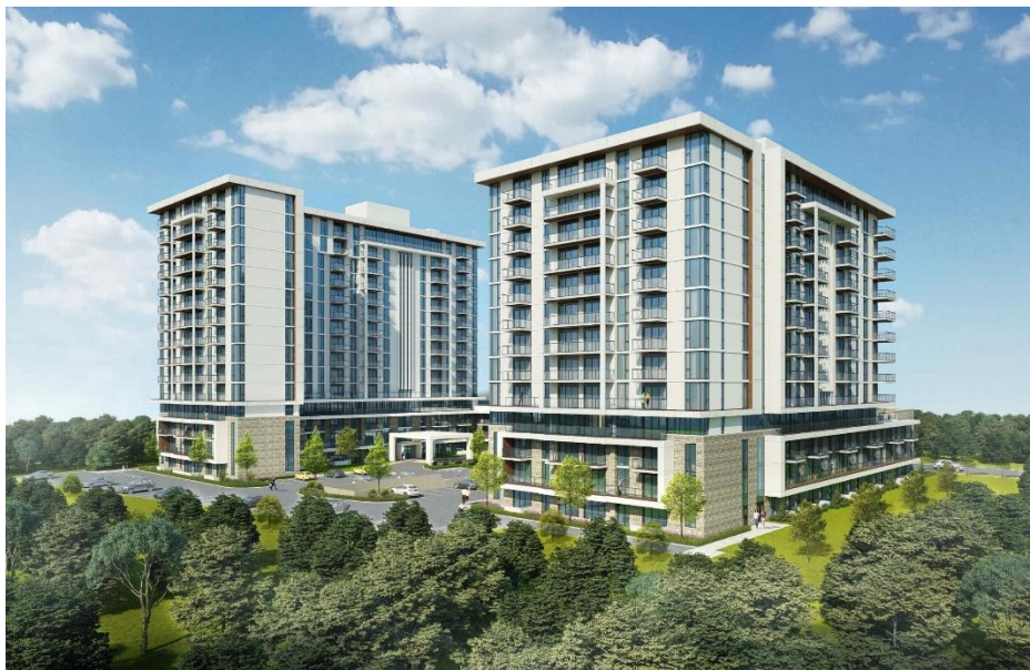
From Rear of Property
