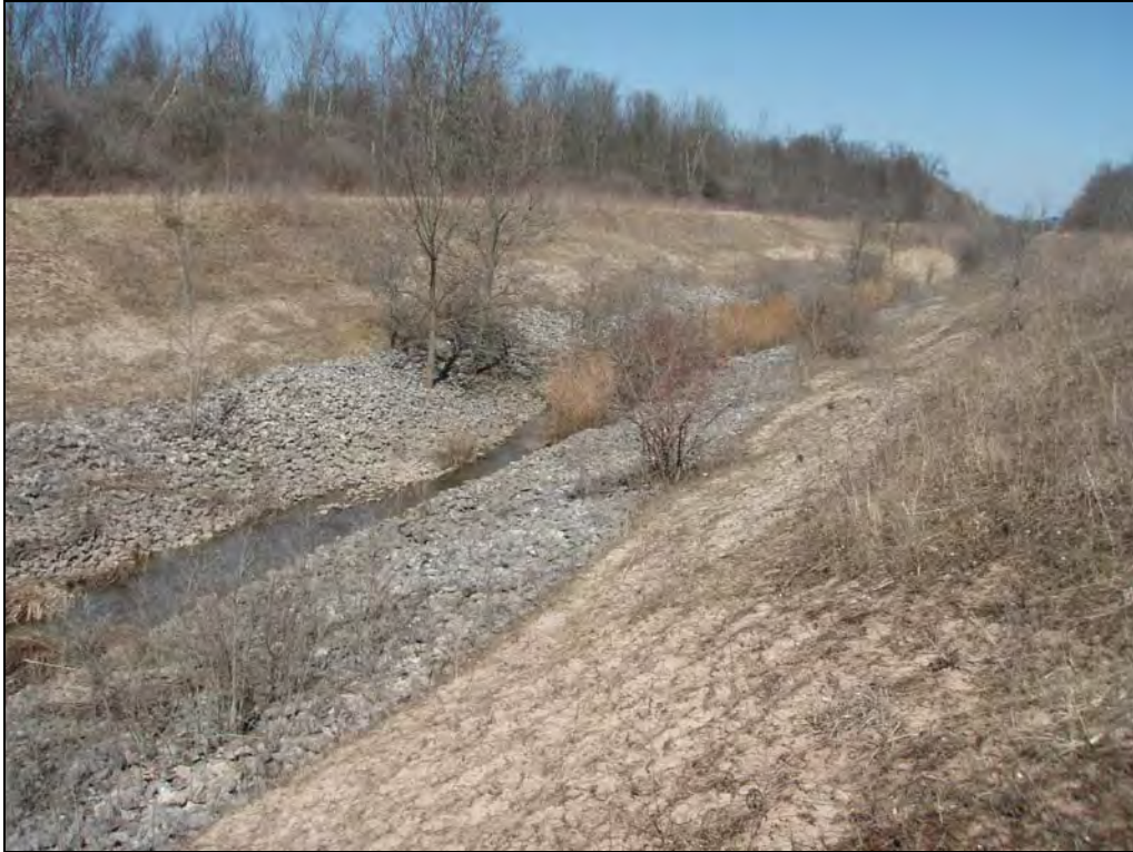
Photograph 10. October 6, 2015. Collapsed rock-filled gabions in sloped section of Watercourse 3, approximately 30 m upstream from mouth.
