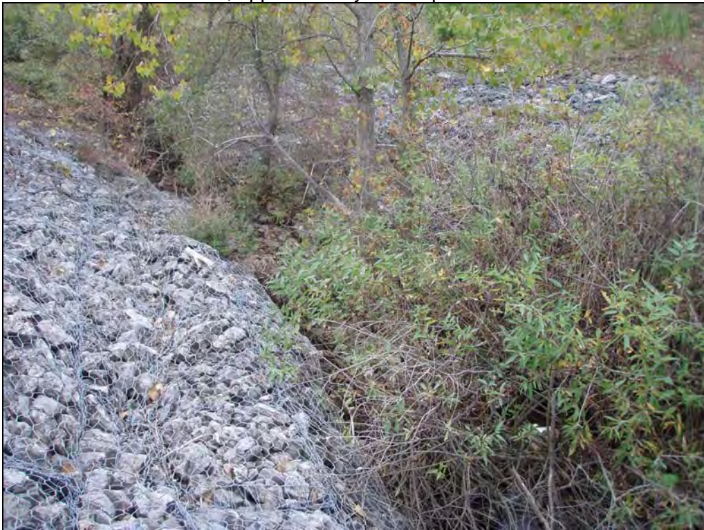
Photograph 10. October 6, 2015. Collapsed rock-filled gabions in sloped section of Watercourse 3, approximately 30 m upstream from mouth.
