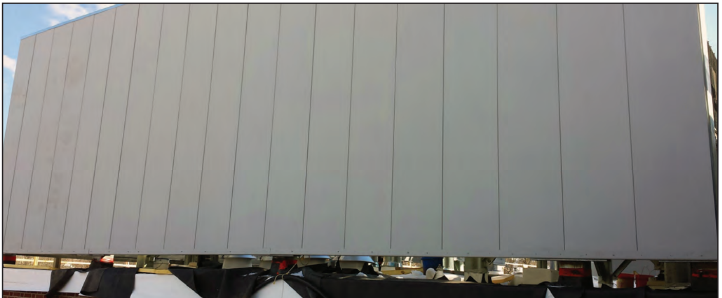
NOISEBLOCK™ rooftop barrier wall surface mounted to structural support steel
