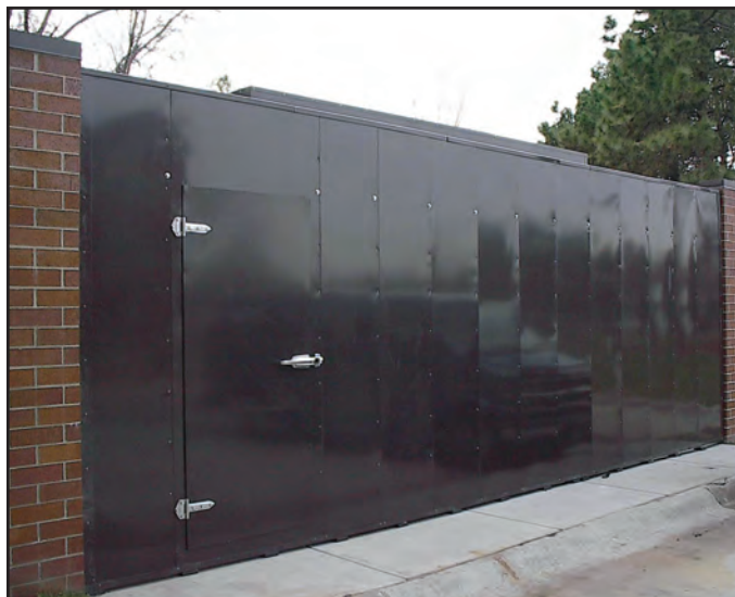
Air-cooled chiller attenuation systems
