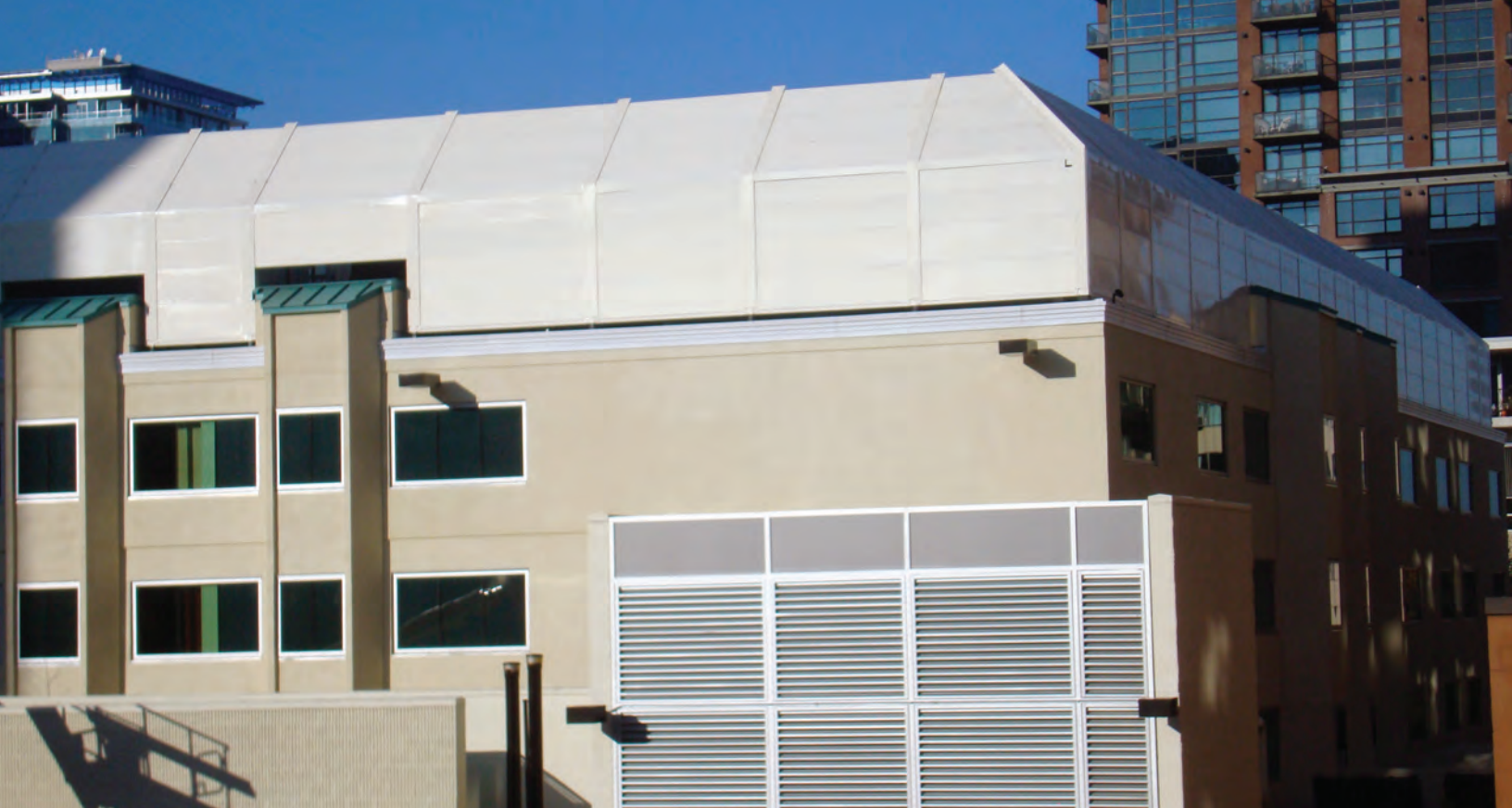
NOISEBLOCK™ wall system, Hospital Rooftop Equipment Yard
