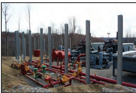
Midstream compressor NOISEBLOCK™ walls
