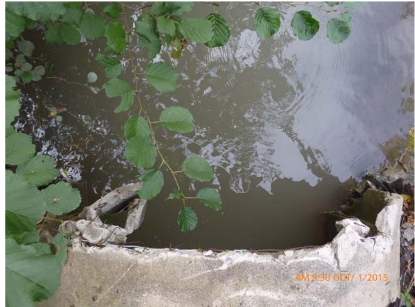
Photo 8: Culvert outlet in state of disrepair.
