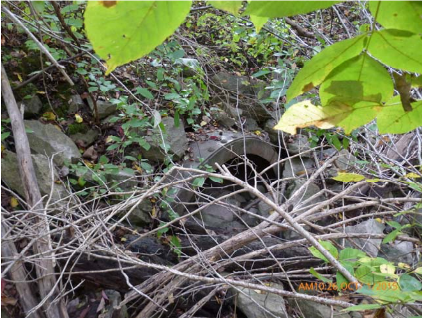
Photo 17: Culvert outlet partially blocked by large rocks.
