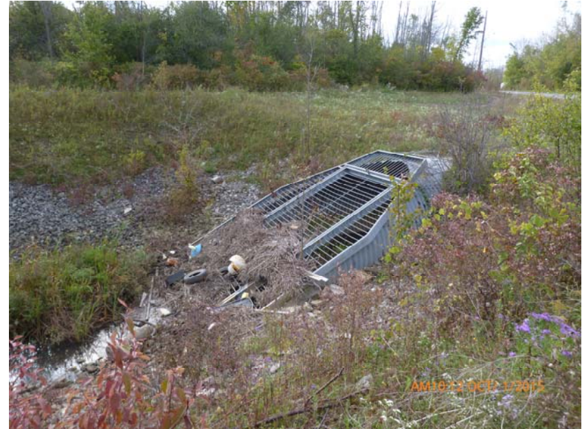
Photo 14: Conrail Drain inlet with safety grate and debris blockage.
