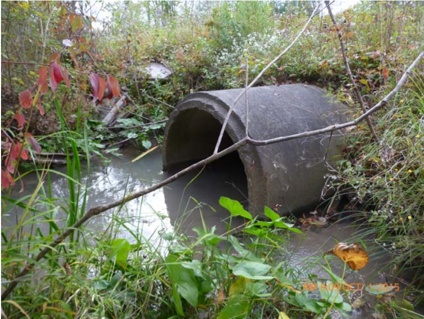
Photo 1: Culvert inlet under the influence of backwater from the Welland River.
