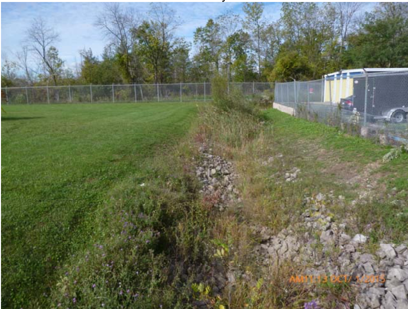
Photo 27: Drainage outlet to power canal.
