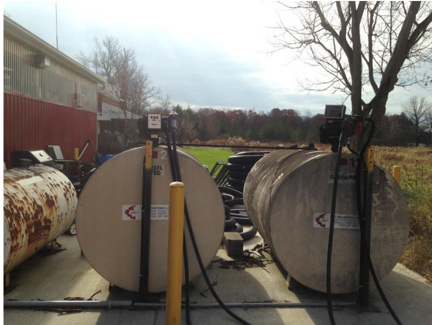
Photograph 5: View of the three ASTs located outside of the smaller barn in the maintenance area located in the central-west portion of the Phase One Property
