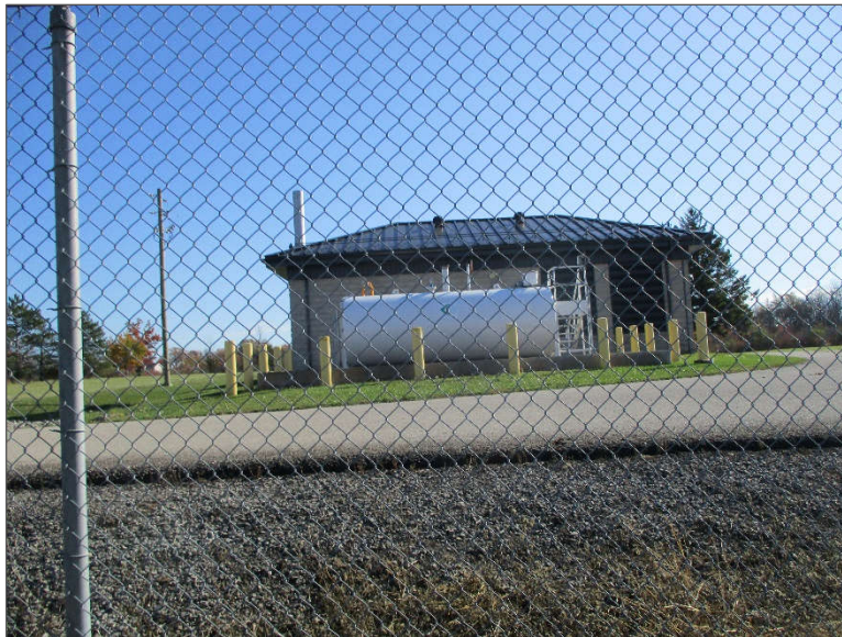
Photo 4 – AST located on the adjacent property to the east of the Site (7606 Oakwood Drive).
