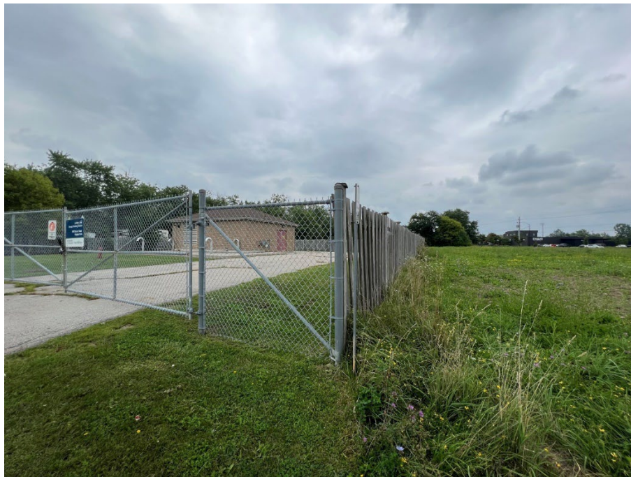
Photo 13 – View looking east of site boundary of Subject Lands (right) with sewage pumping station (left).
