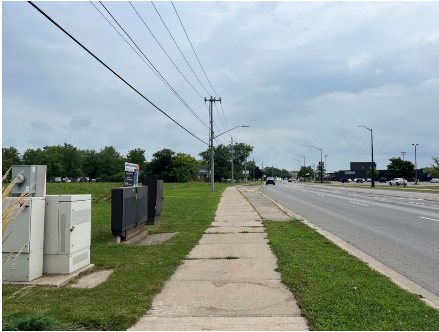
Photo 6 – View toward west-northwest of Subject Lands and utility boxes (left) and Lundy's Lane (right).
