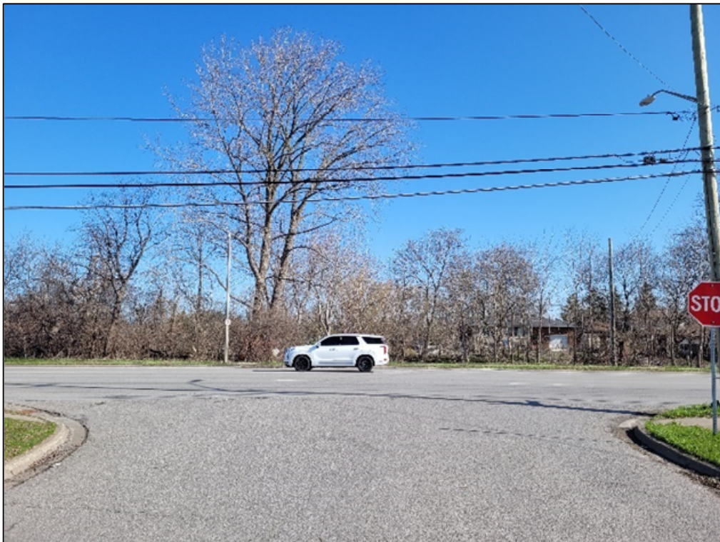
Figure 3 - Subject Lands, Looking North from Collard Avenue
