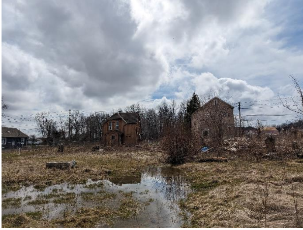
Photo 1: View of subject site from Northern boundary
