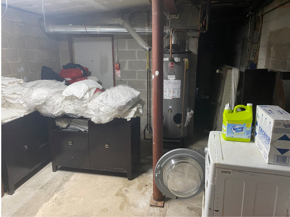
Photo 5: Storage Room (looking W).
