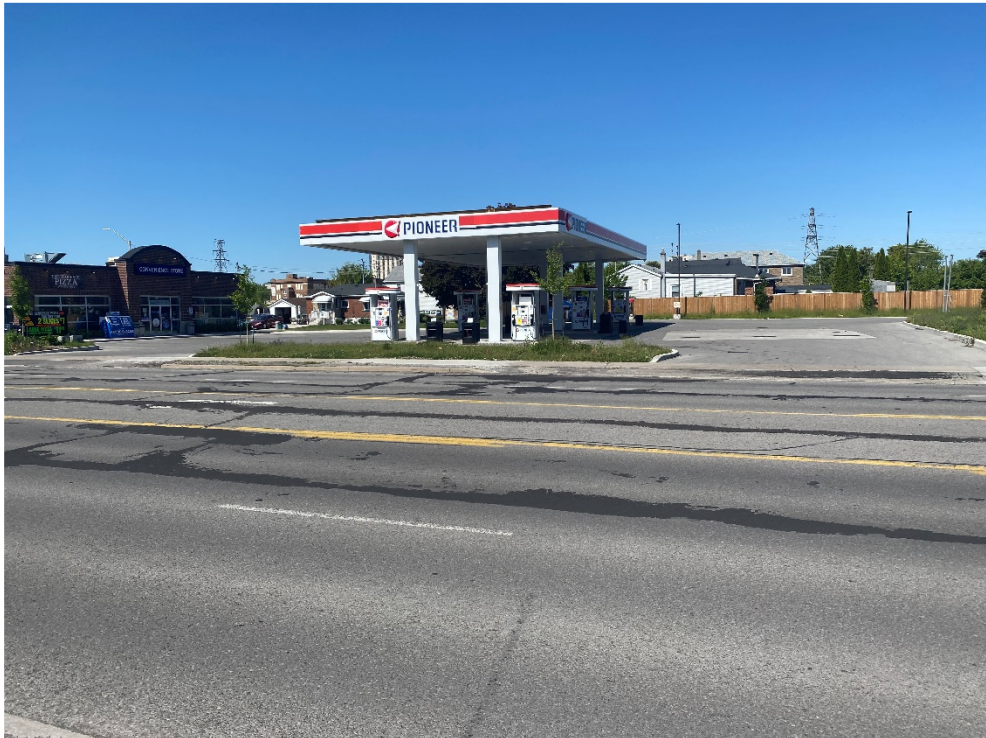
Photo 16: Adjacent Commercial Property to West (looking W).
