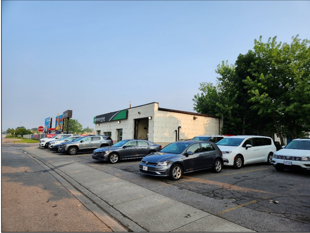
Figure 4 - 5590 Stanley Avenue - Enterprise Car Rental - Northeast Corner of Stanley Avenue and North Street
