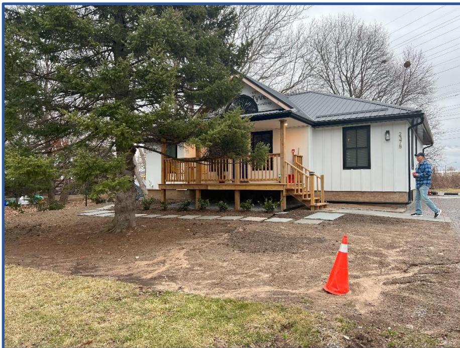
Photo 10 – View toward the southeast of 2378 Portage Road from sidewalk.
