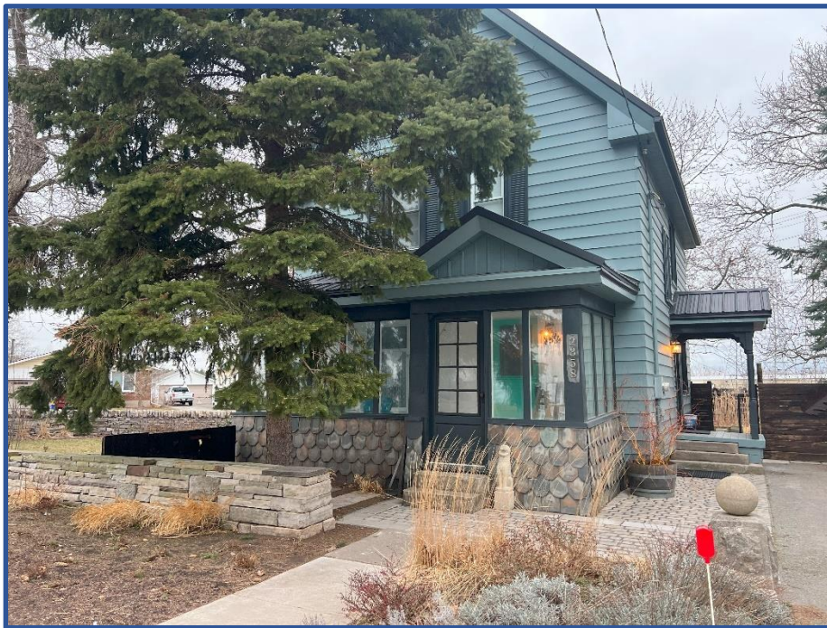
Photo 4 – View of two-and-a-half storey detached dwelling on 2358 Portage Road, looking southeast.
