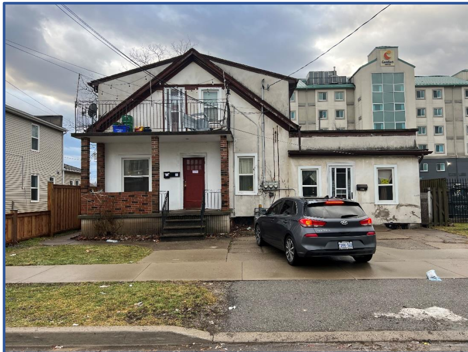
Photo 2 – View of triplex dwelling neighbouring Subject Lands to the north and looking west from Buchanan Street. Comfort Hotel is visible in the background.
