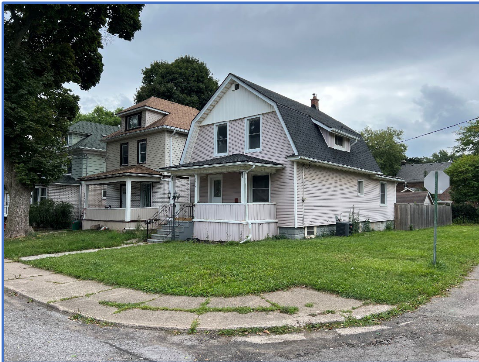
Photo 2 – View of 5014 Willmott Street, looking southeast from intersection of Willmott Street and Third Avenue.
