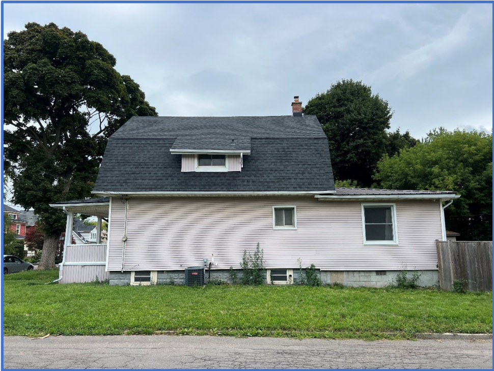
Photo 3 – View of 5014 Willmott Street, looking east from Third Avenue.
