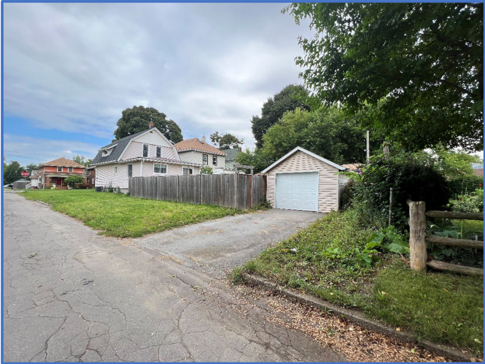
Photo 4 – View of the driveway and detached garage located at the rear of the Subject Lands and accessed from Third Avenue.
