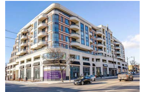
Figure 33: Example of Apartment Residential
