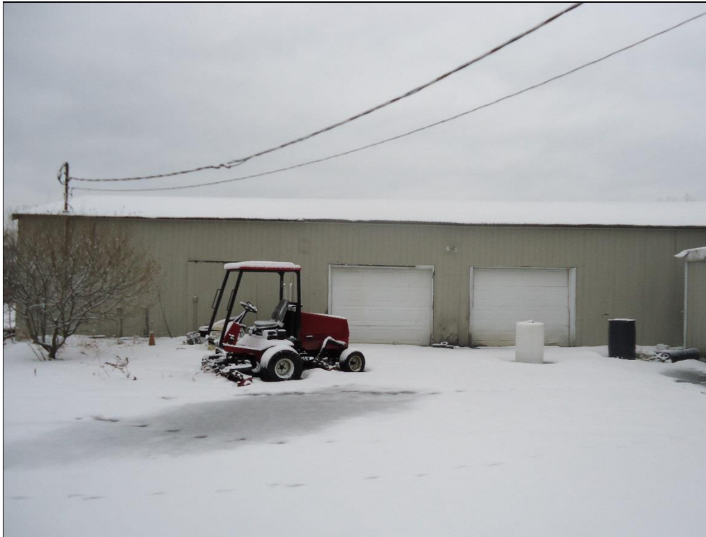
Photo 3: Maintenance equipment storage warehouse.
