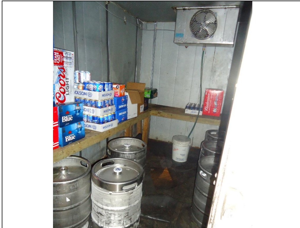
Photo 7: Walk-in cooler adjacent to kitchen Date: January 24, 2019 Direction: -
