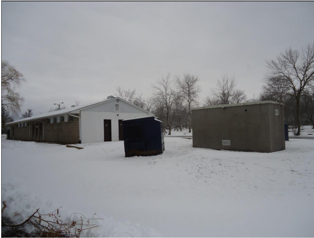
Photo 5: Washroom/shower/ laundry facilities building and sewage pump house building.
