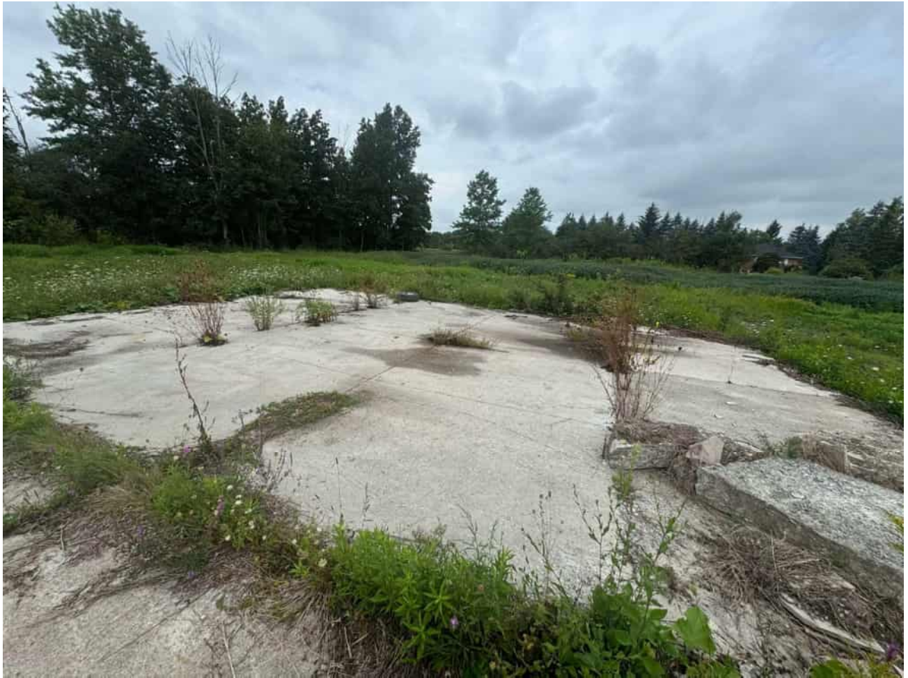
Photograph 2: Remaining concrete pad foundation of the garage. Limited staining was noted.
