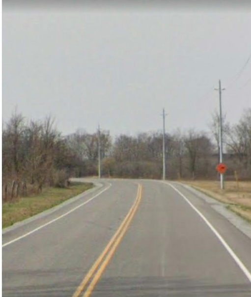
Figure 1-3 Looking West along Chippawa Ck. Rd.
