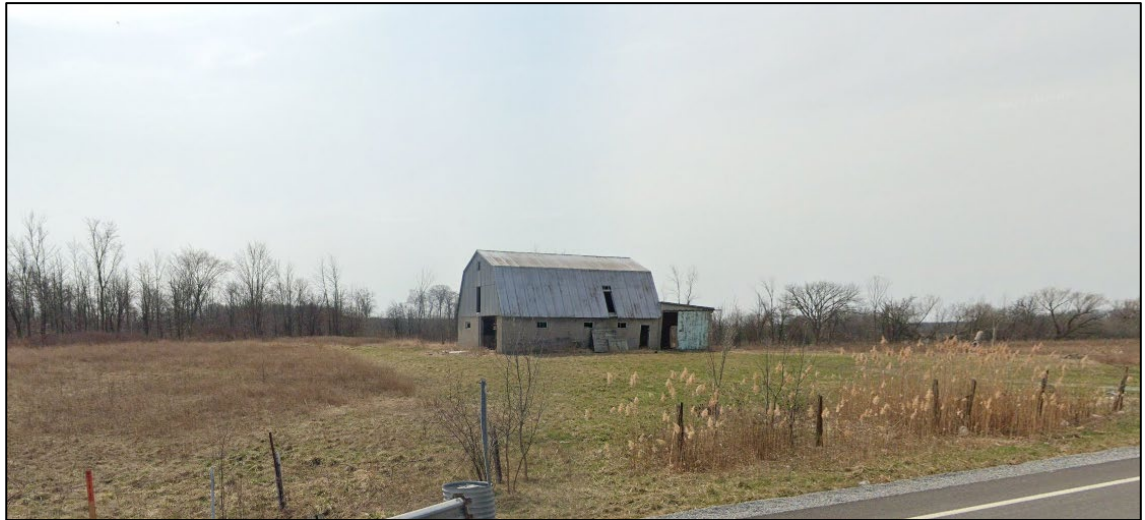
Figure 3-3: View of Barn Structure along Chippewa Creek Road, Retrieved from Google Streetview
