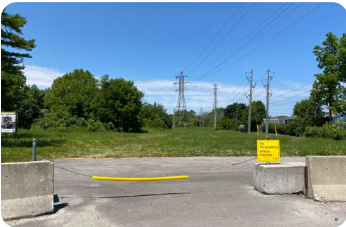
View of hydro corridor to west of site
