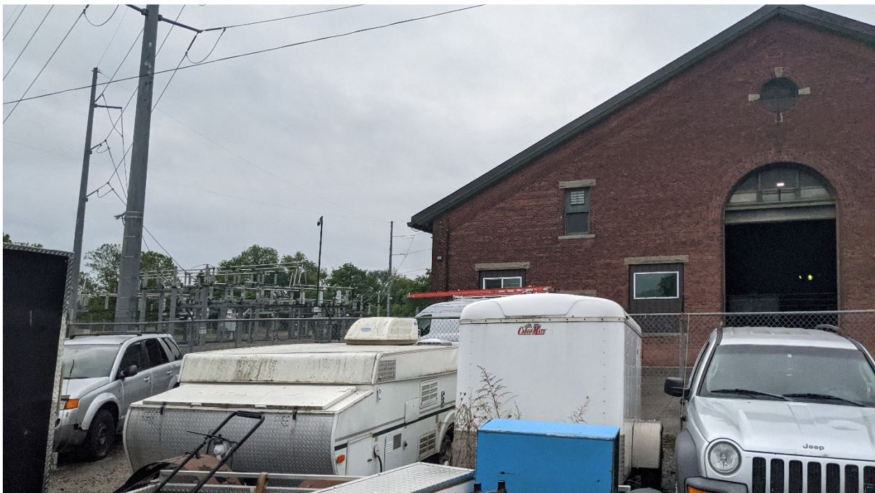
A view of the adjacent hydro station and hydro transformers, from the south end of the Site, facing southeast.
