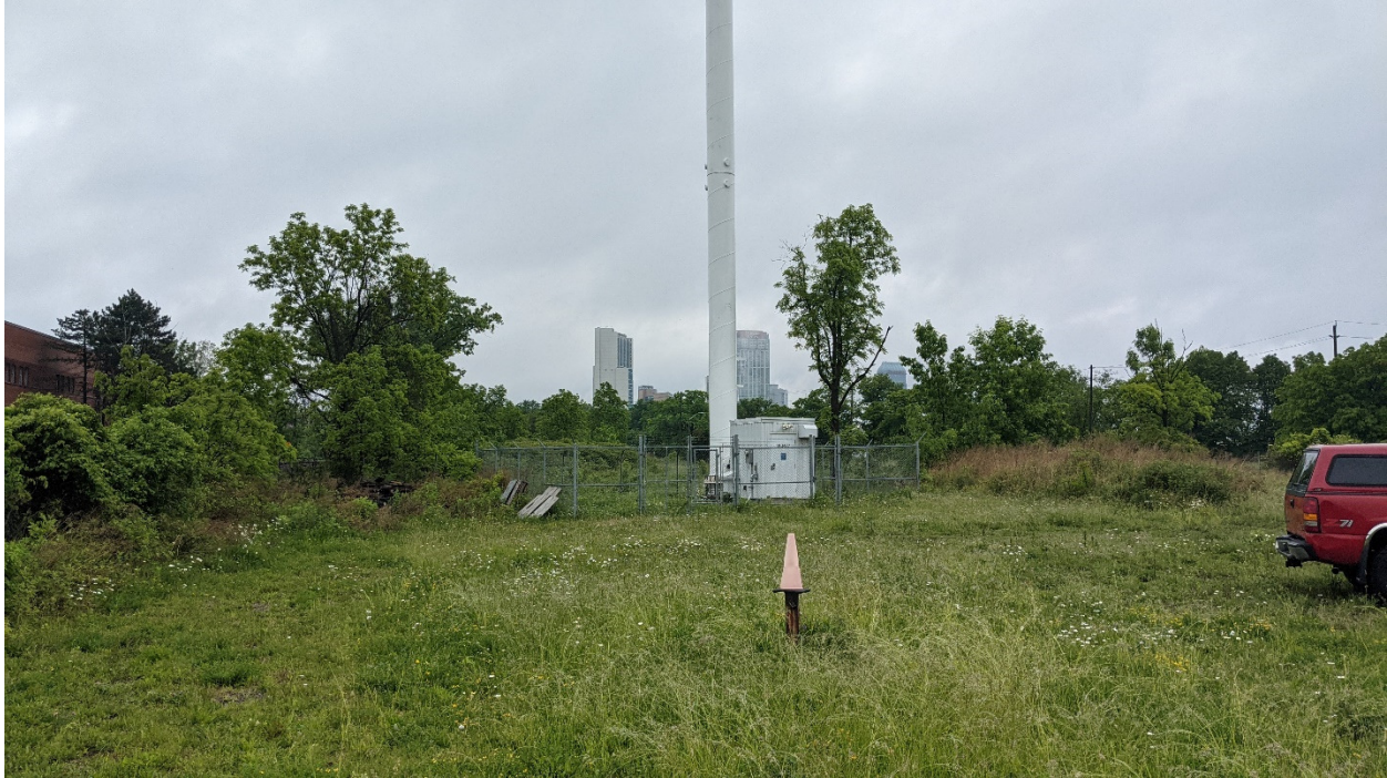
West end of the Site, facing northwest. The on-site monitoring well is visible on the bottom of the photo with the on-site communication tower in the background.
