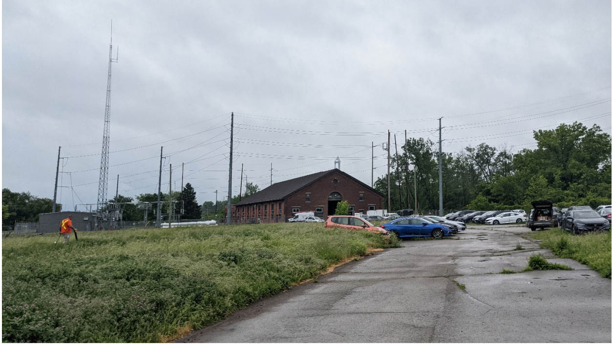
Photo from the east end of the Site, facing south with the adjacent hydro station visible in the background.
