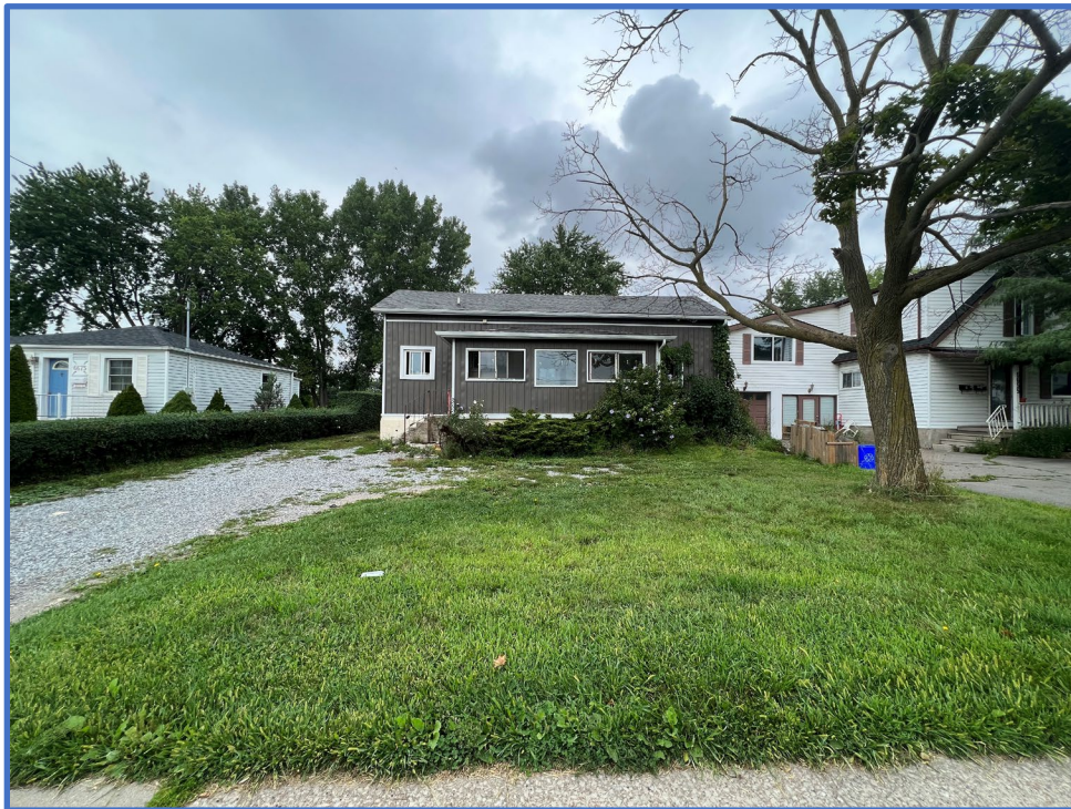
Photo 4 – View of 6665 McLeod Road, looking north.
