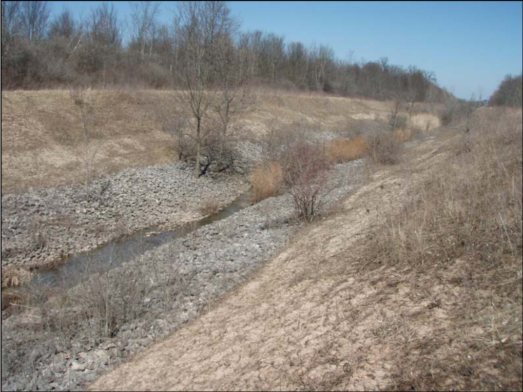
Photograph 9. April 12, 2015. Structure of Watercourse 3.
