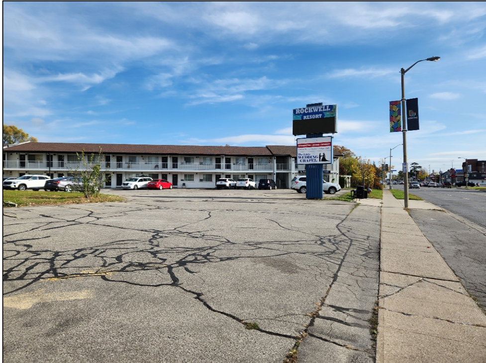
Figure 2 - Area of the subject lands where the 6-storey apartment building will be located. The driveway entrance shown in this photo will be removed.
