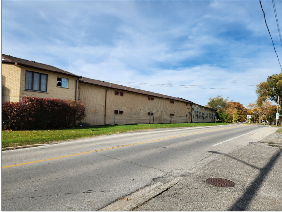
Figure 4 - The easterly facade of the building, viewed from Beaverdams Road
