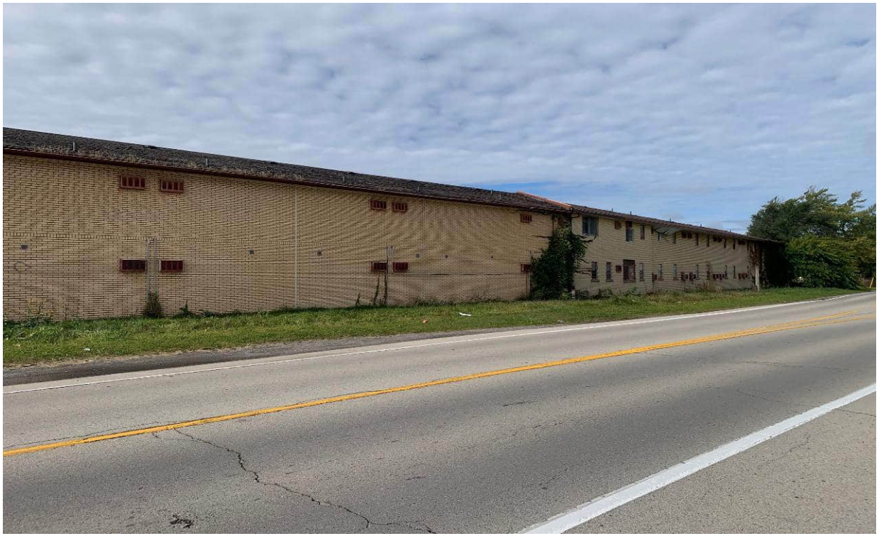
Photograph No.3 – Exterior east side.
