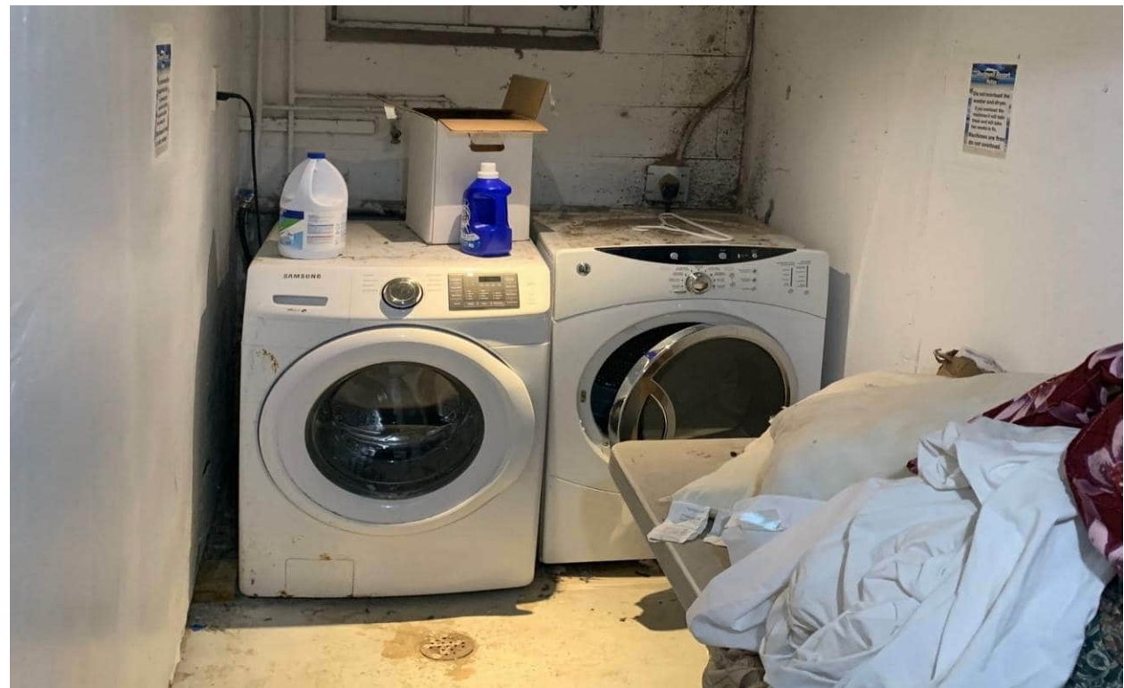
Photograph No.12 – Laundry room.
