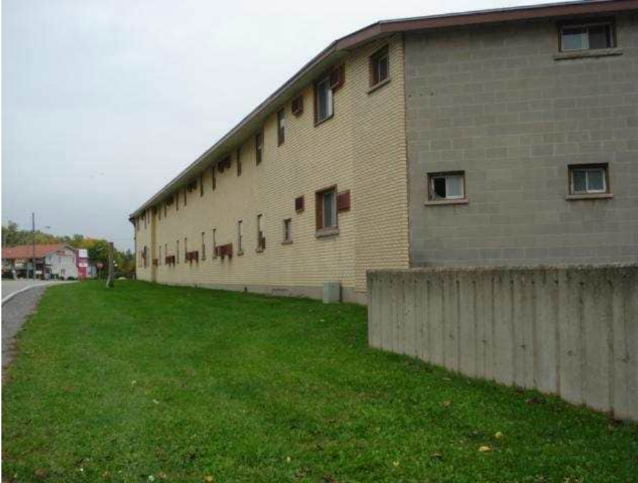
Rear of East Section
