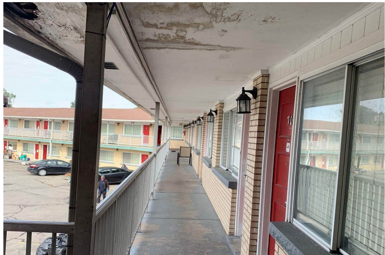
Photograph No.16 – Potential lead-based paints.
