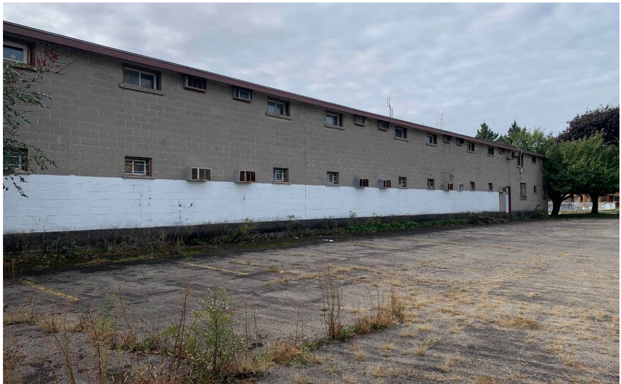
Photograph No.2 – Exterior north side.
