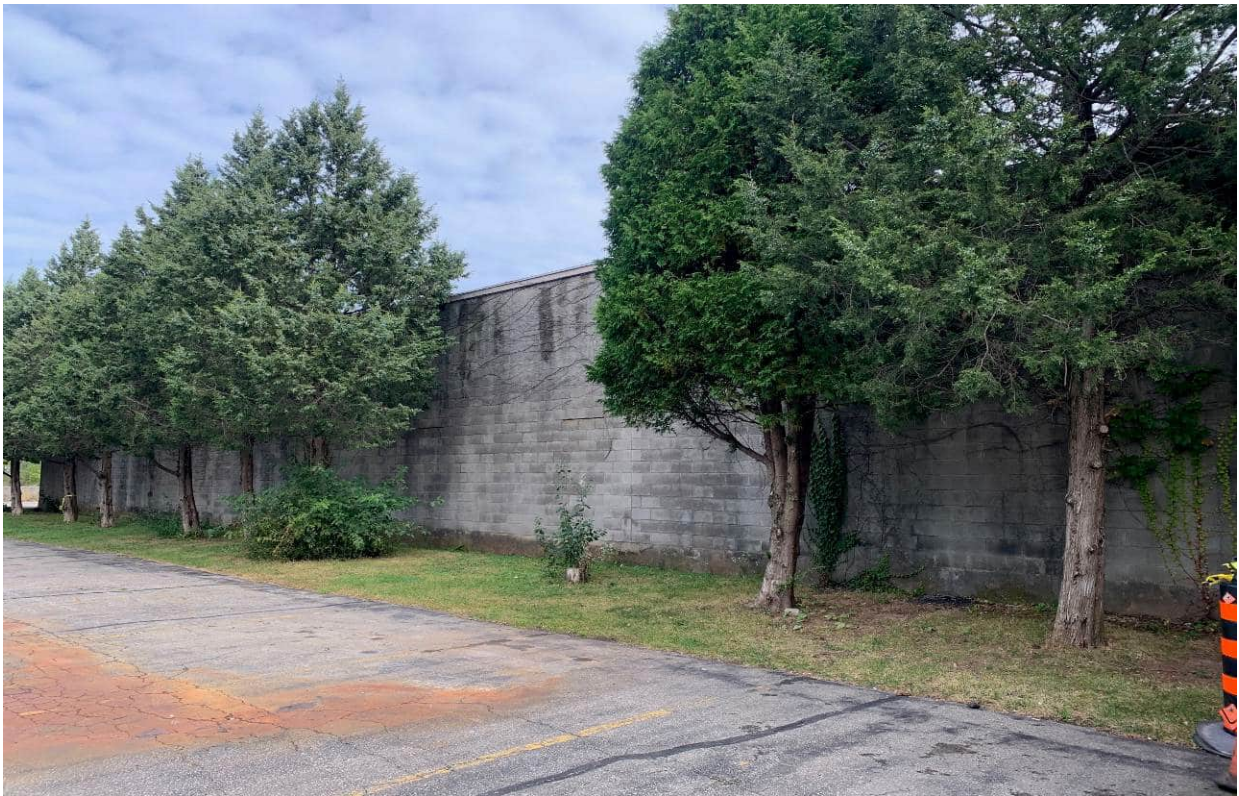
Photograph No.4 – Exterior west side.
