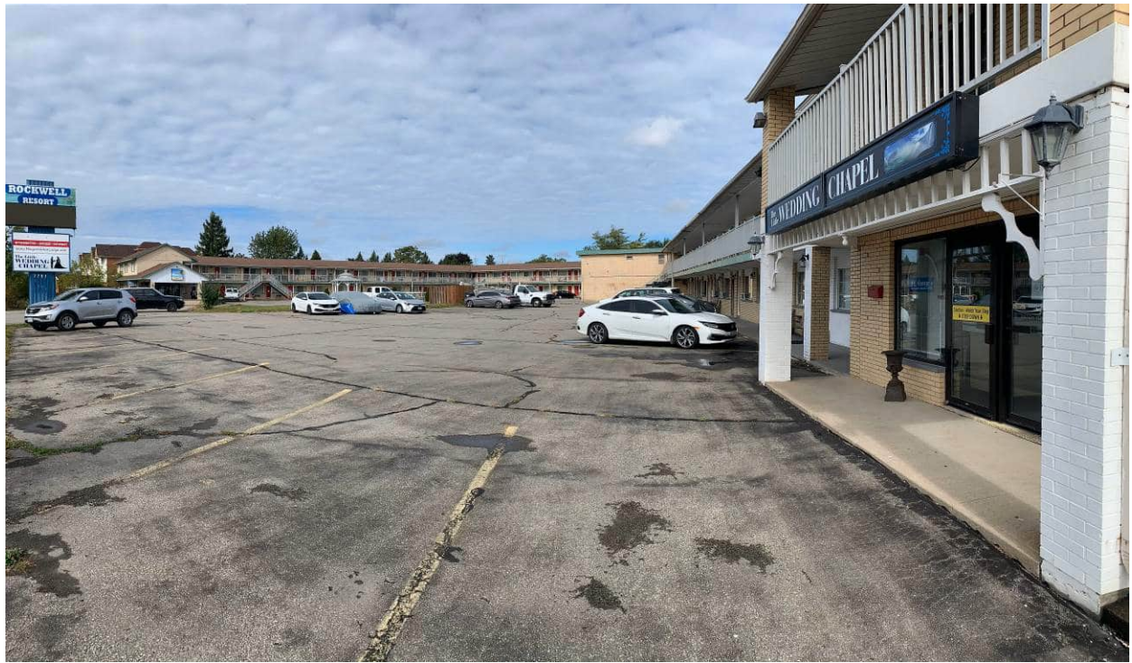
Photograph No.1 – Exterior south side.
