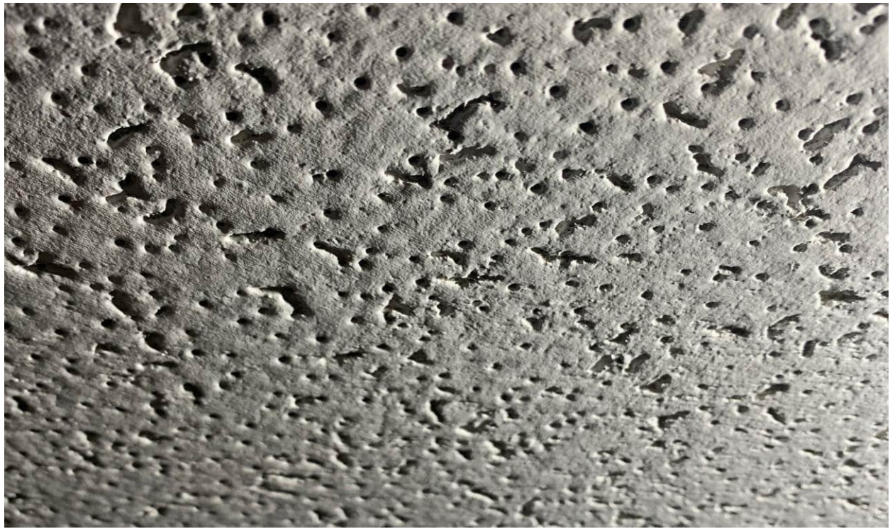
Photograph No.13 – Ceiling tiles.
