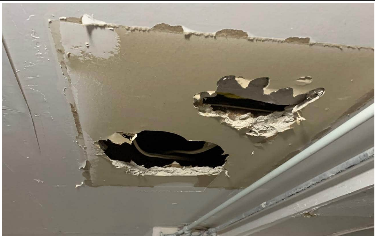
Photograph No.14 – Basement ceiling, drywall joint compound.
