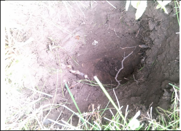
IMAGE 2 COMPLETED TEST PIT
