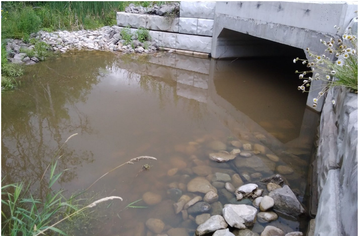
Figure 6: Culvert downstream of the Cattail Marsh
