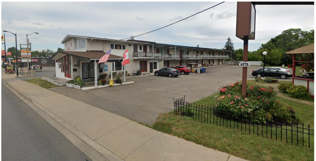
Figure 3 – Street View of Subject Property from Lundy's Lane (east of motel)
