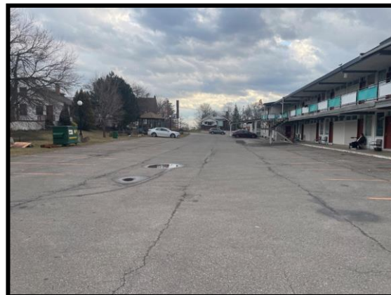
Image 10: Area of Potential (February 9, 2024; Facing Southeast)
