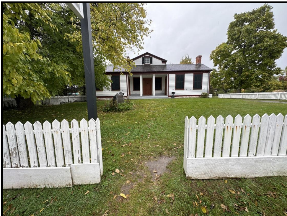
Image 36: Façade of 6137 Lundy's Lane from Sidewalk (Photo taken on October 20, 2023; Facing North)
