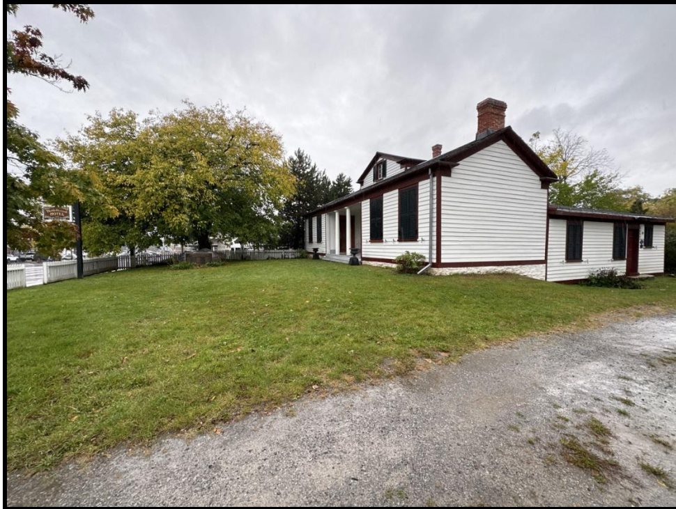
Image 39: 6137 Lundy's Lane – East Elevation (Photo taken on October 20, 2023; Facing West)
