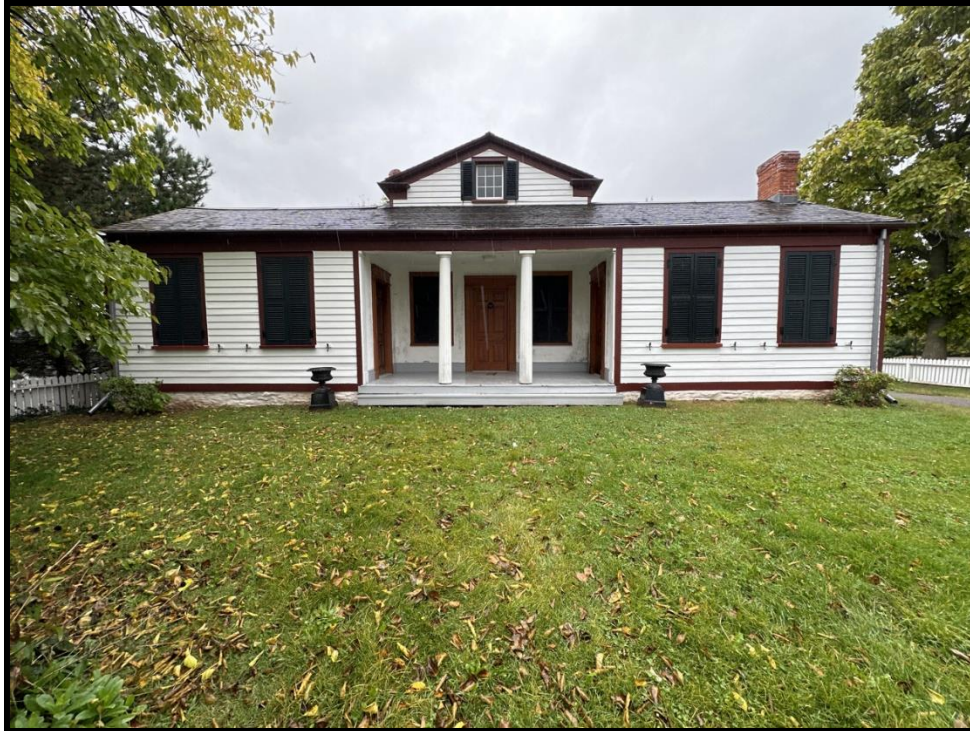
Image 37: 6137 Lundy's Lane – Façade (Photo taken on October 20, 2023; Facing North)
