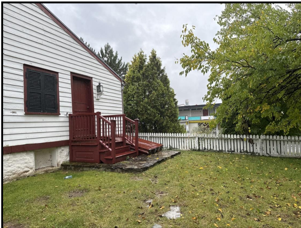
Image 40: 6137 Lundy's Lane – Rear Elevation (Photo taken on October 20, 2023; Facing West)
