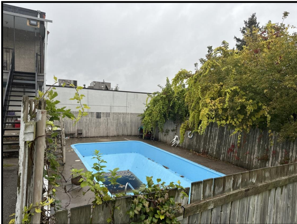
Image 20: Subject Property at 6179 Lundy's Lane – Pool at Rear of Motel (Photo taken on October 20, 2023; Facing Northwest)
