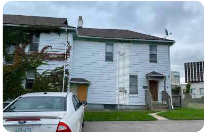
Subject Lands - Listed Heritage Property Looking East
