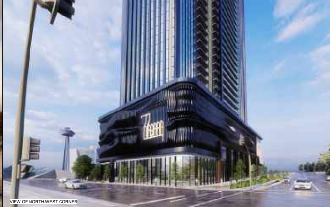
VIEW OF NORTH-WEST CORNER
