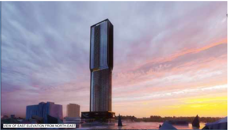
VIEW OF EAST ELEVATION FROM NORTH-EAST
