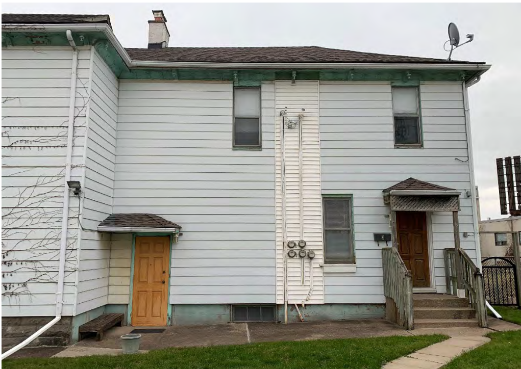
Plate 34 View of the southern portion of the west elevation, facing east.
