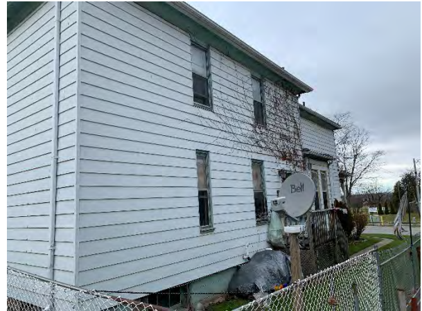
Plate 38 View of the south portion of the east elevation showing the modern wooden deck structure, facing north-northwest.
