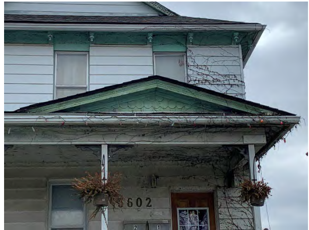
Plate 29 View of decorative pediment on the front porch, facing south.
