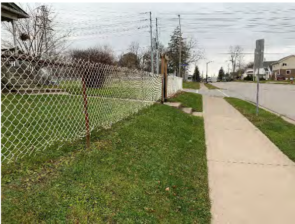
Plate 20: View showing the raised grade of the Study Area along Robinson Street, facing east.
