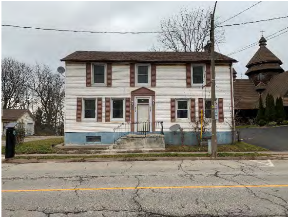
Plate 12: South elevation of 6214-6218 Main Street (listed heritage property).
