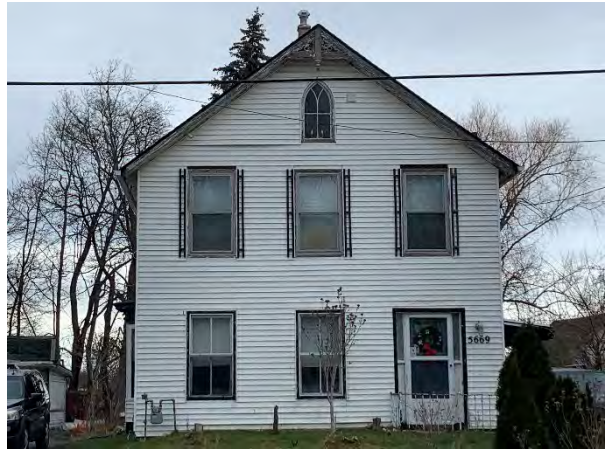
Plate 9: South elevation of 5669 Robinson Street (listed heritage property).
