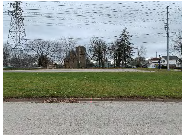
Plate 7: View of designated All Saints Church (5680 Robinson Street; designated under Part IV of the Ontario Heritage Act ) from the Study Area, facing west.
