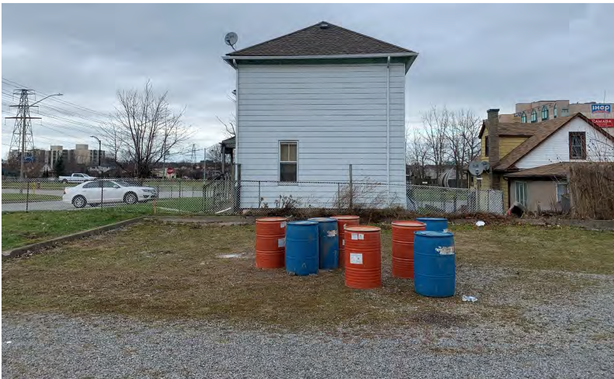
Plate 17: South elevation of 5602 Robinson Street
