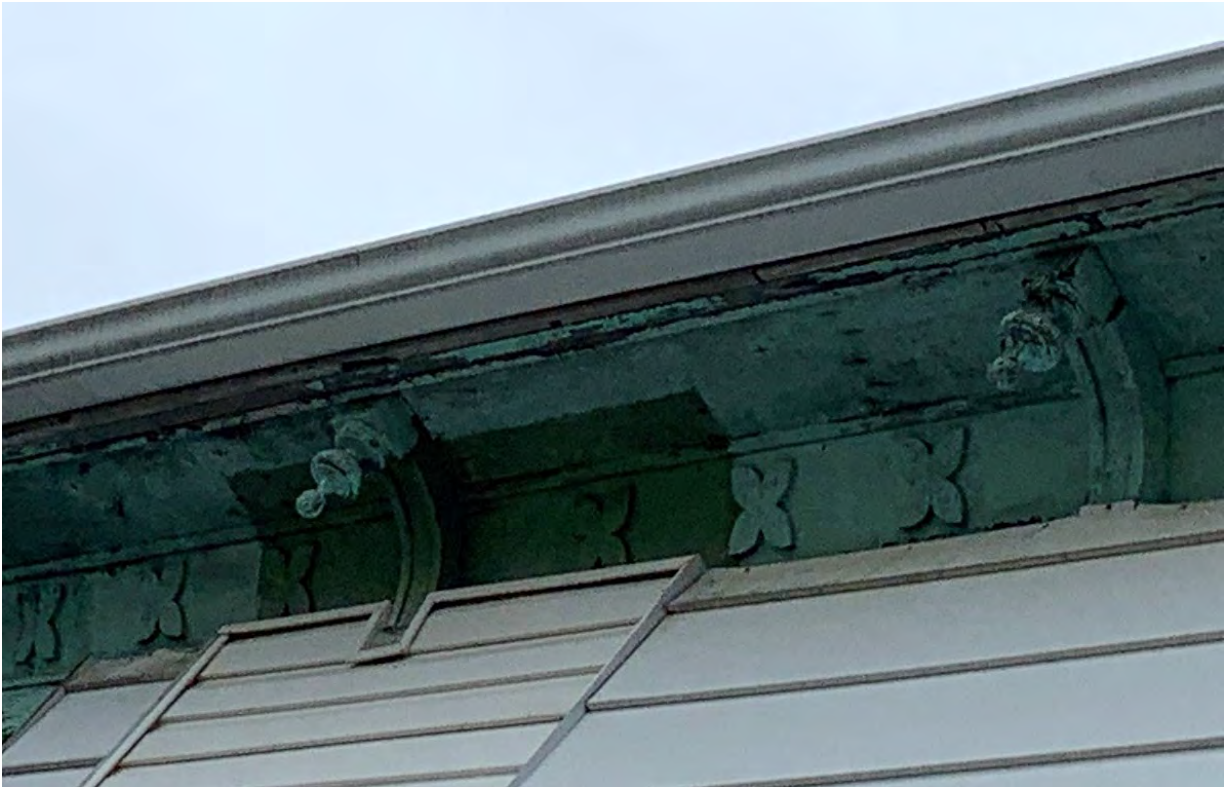
Plate 35 View of the decorative motif below the eave in the section of the west elevation that has been retrofitted with aluminium siding, facing east.
