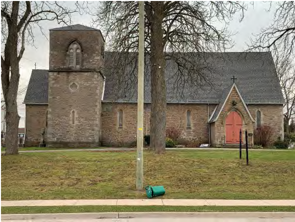
Plate 8: North elevation of All Saints Church (5680 Robinson Street; designated under Part IV of the Ontario Heritage Act ).
