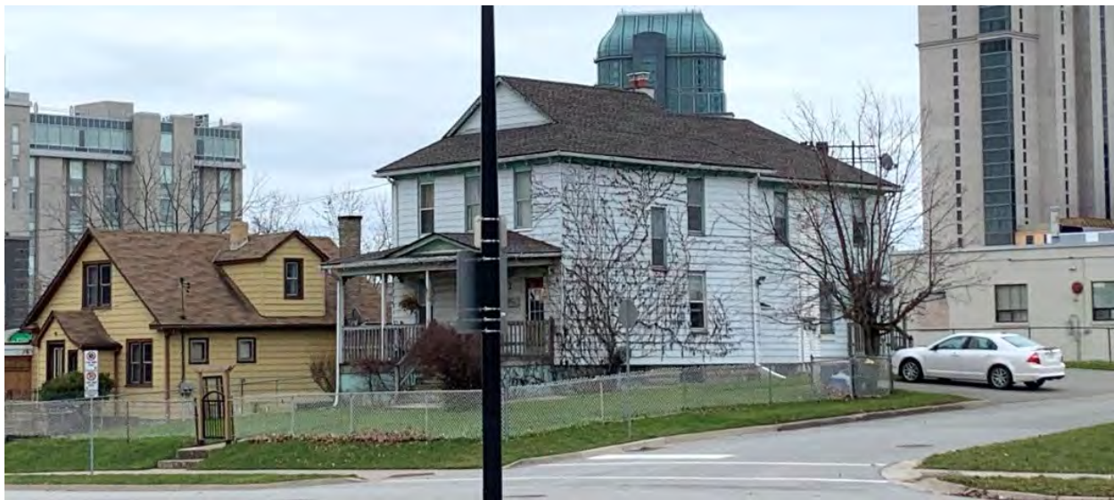
Plate 1: Oblique view of 5602 Robins Street from the northwest corner of Robins Street and Allendale Avenue, facing southeast.
