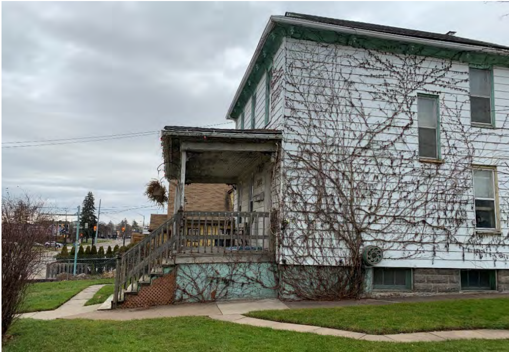
Plate 33 View of the north section of the west elevation, facing east.
