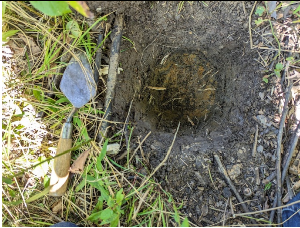
Photo 9: Typical test pit
