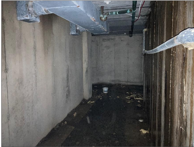
Photo 17 – View of unfinished basement in the vicinity of the inground pool.
