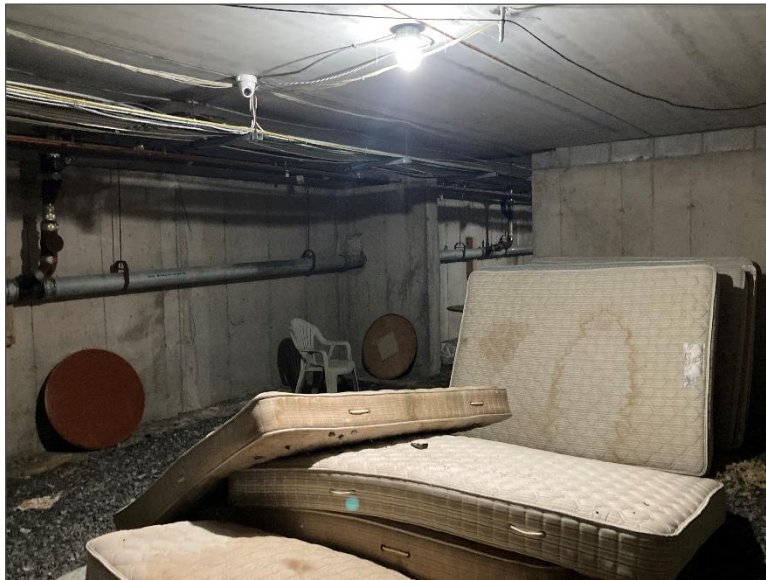
Photo 18 – View of the north portion of the unfinished basement.
