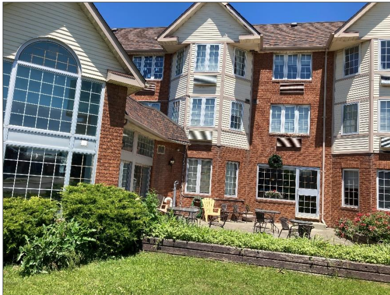
Photo 2 – Site Building (partial south elevation).
