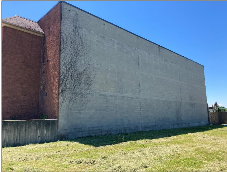
Photo 1 – Site Building (north elevation).
