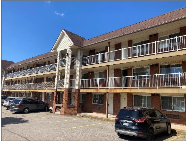
Photo 3 – Site Building (partial east elevation).
