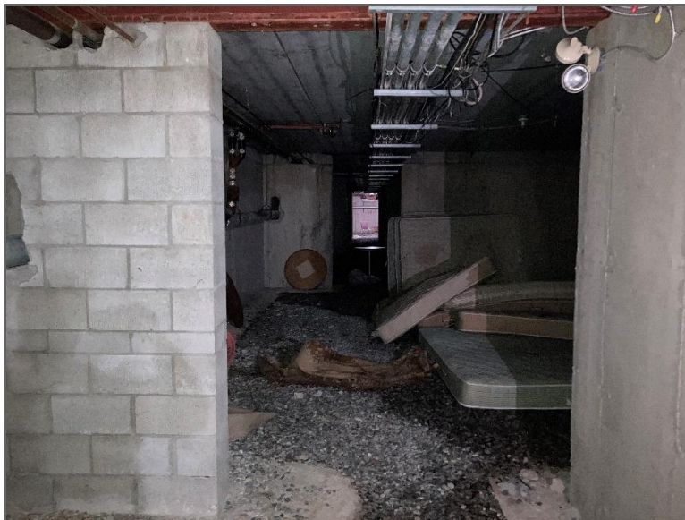
Photo 14 – View of north portion of unfinished basement.
