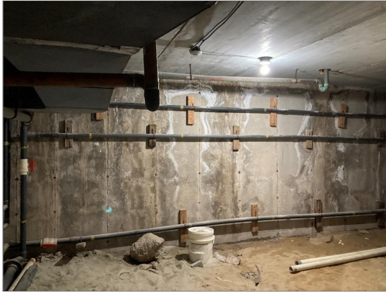
Photo 13 – View of exterior concrete wall of indoor swimming pool.
