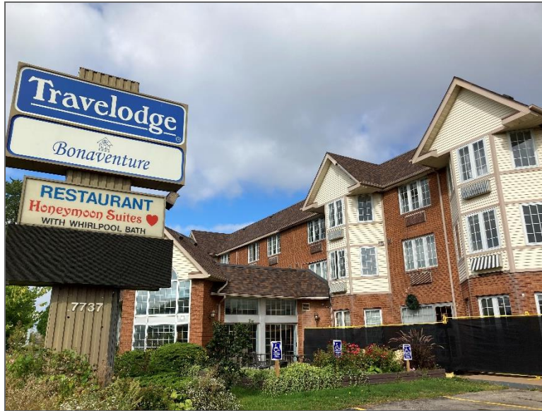
Photo 1 – South elevation of the Site Building, looking northwest.
