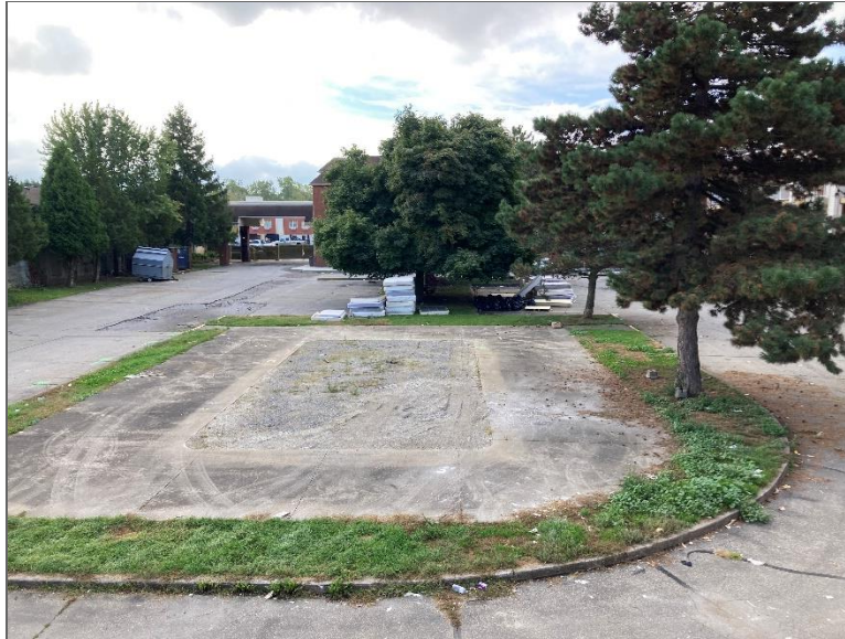
Photo 9 – Exterior infilled swimming pool located on the central portion of the Phase One Property
