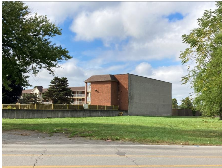
Photo 2 – North elevation of the Site Building, looking southwest.
