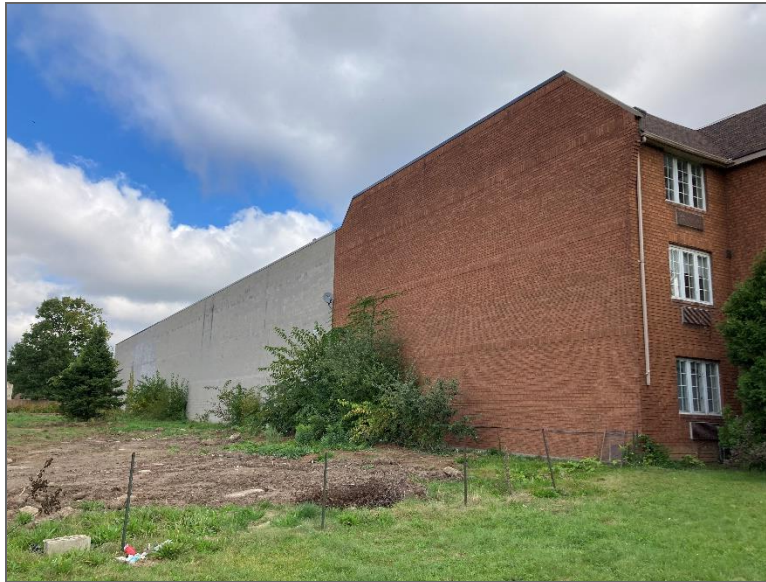
Photo 3 – West elevation of the Site Building, looking northeast.
