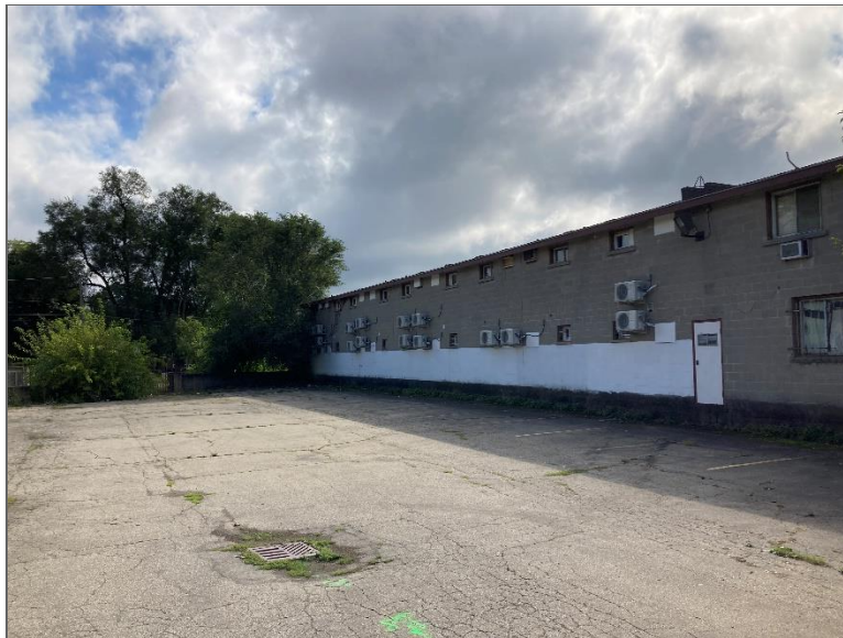
Photo 8 – Rear portion of property building located west of the Phase One Property.
