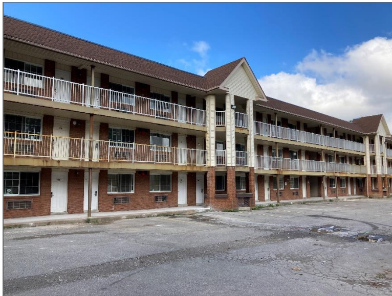
Photo 4 – East elevation of the Site Building, looking northwest.
