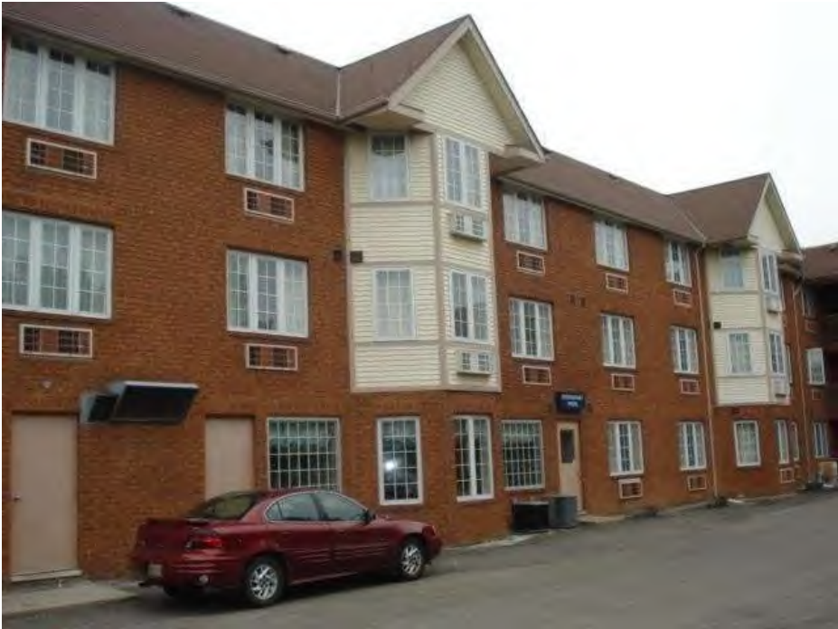
Rear of Hotel Section
