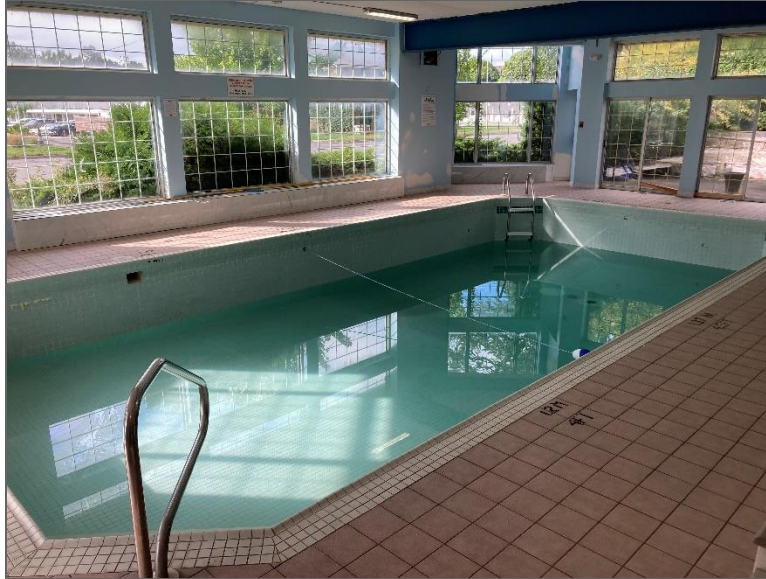
Photo 15 – View of indoor swimming pool on main floor of Site Building.
