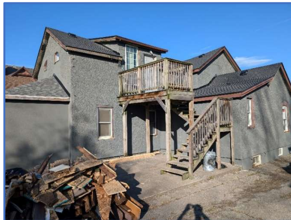
Photo 2 – External staircase, providing access to the second-floor unit
