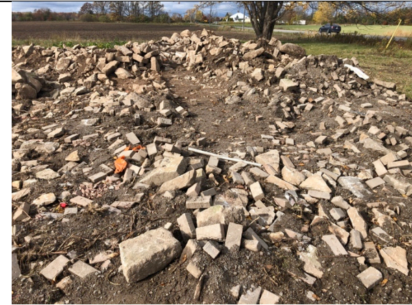
IMAGE 4 DEBRIS PILE FROM DEMOLITION OF HOUSE
