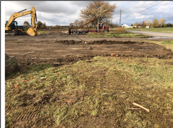
IMAGE 1 REMOVAL OF TOPSOIL WHERE HOUSE WAS PREVIOUSLY LOCATED
