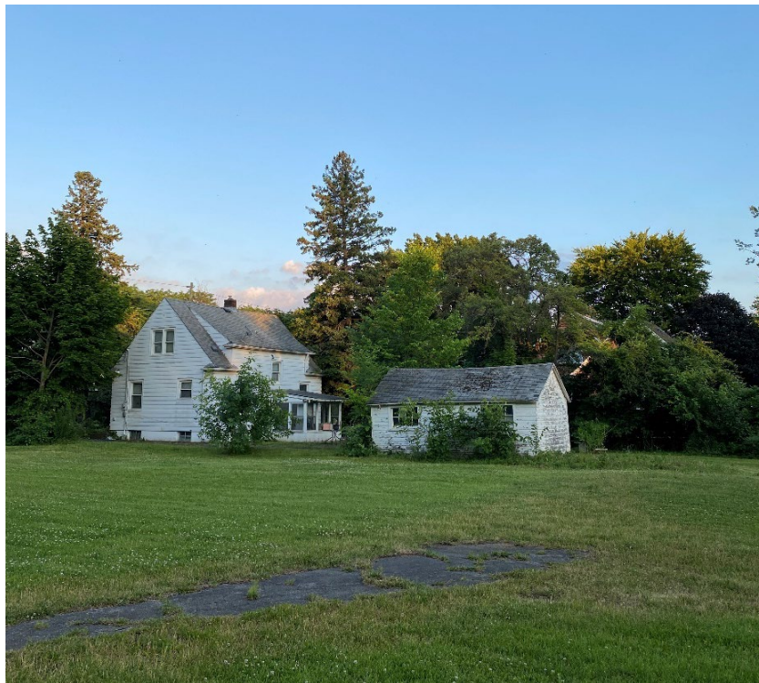
Photo 2: Outbuilding 1, located in close proximity to the single-family residence at 6393 Dorchester Road.
