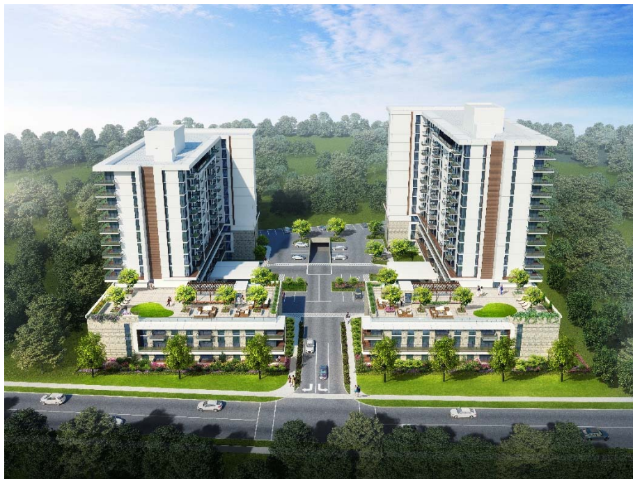
APARTMENT DEVELOPMENT LOOKING EAST
