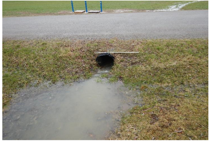
Photo 2: April 4, 2017 - Feature 1. At Uppers Lane facing downstream (north)
