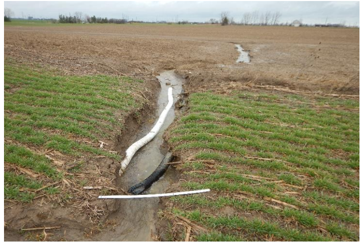
Photo 14: April 4, 2017 - Feature 4. Exposed tile drain. Facing downstream (northwest) at field crossover
