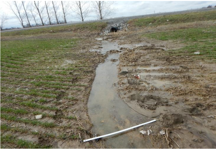
Photo 33: April 4, 2017 - Feature 10. At upstream section facing upstream (west)
