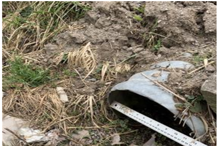
Photo 76: April 9, 2021 – Feature 18. Uppers Lane culvert
