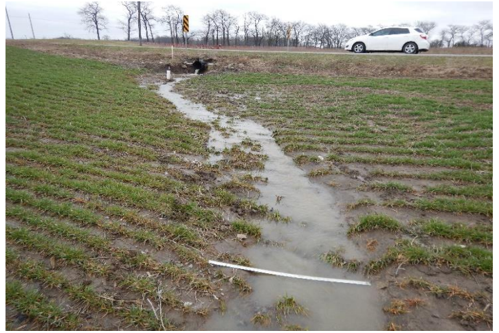
Photo 44: April 4, 2017 - Feature 13. At upstream section facing upstream (south)
