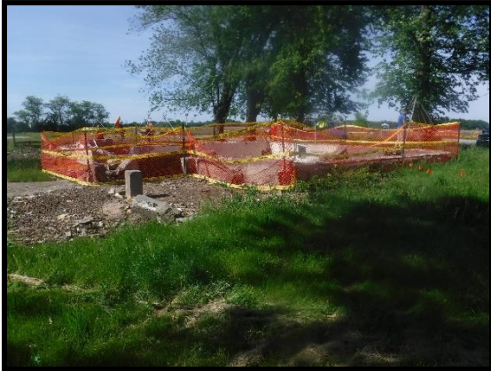
Image 1: Field Conditions (June 12, 2019; Facing Southwest)
