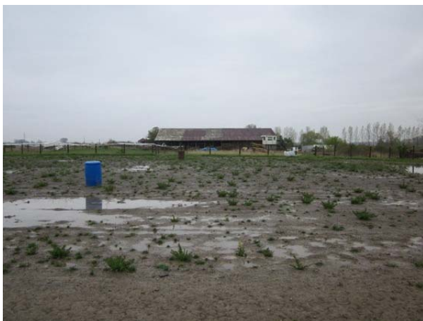
Plate 35. #9903 Uppers Lane Farm Complex (Rear) (view south)
