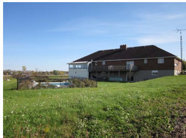
Plate 30. #5205 Beechwood Rd. Residence (Rear) (view northeast)
