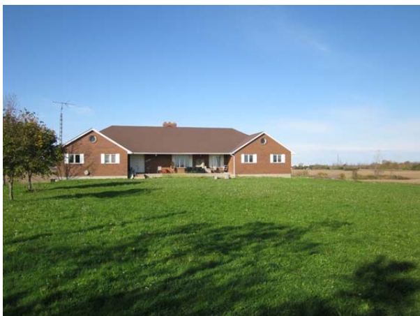
Plate 29. #5205 Beechwood Rd. Residence (Front) (view west)
