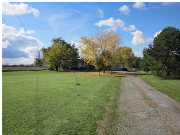
Plate 36. #5545 Beechwood Rd. Residence (Front) (view west)
