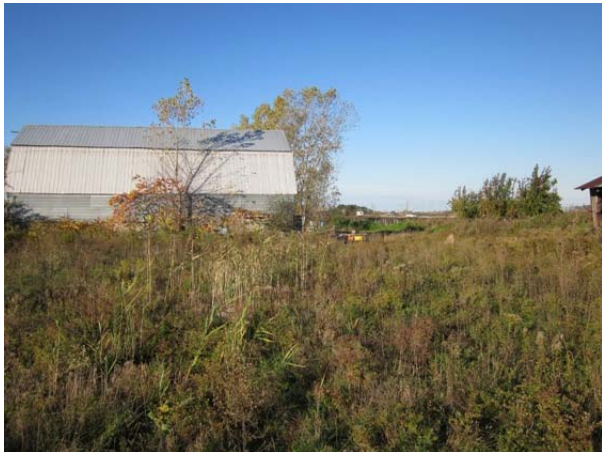
Plate 27. #9903 Uppers Lane Farm Complex (view west)
