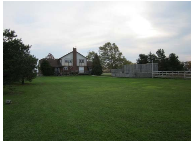
Plate 40. #5497 Beechwood Rd. Residence (Rear) (view east)
