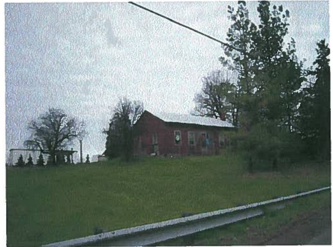
Plate 4: Looking northeast at historic house located at 10033 Upper's Lane.
