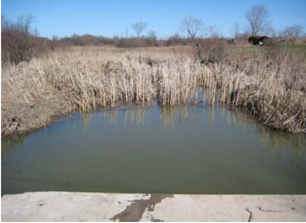
Photograph 5 ↑ North pool at Uppers Lane culvert
