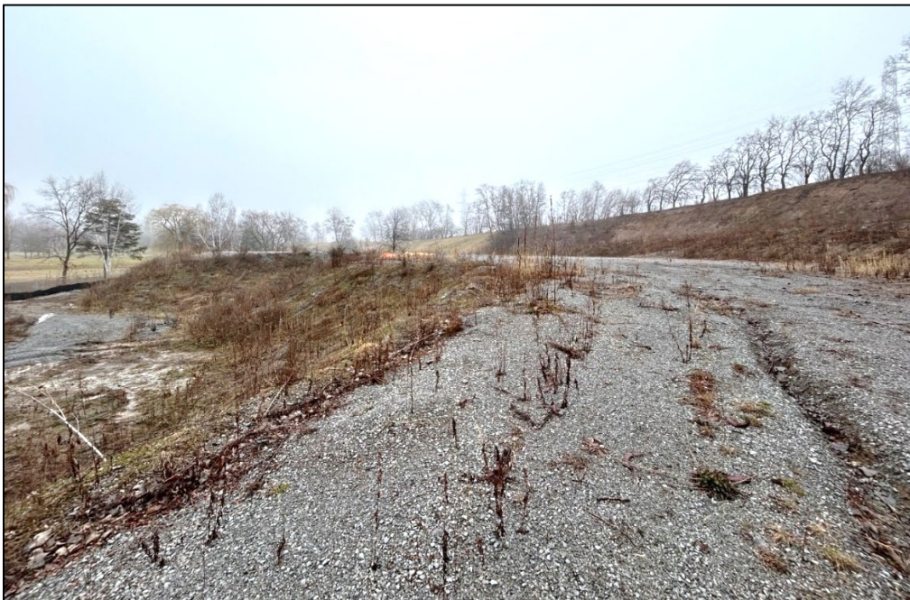
Figure 4 - View of built-up grade at centre on Subject Lands with Mountain Road at highest grade to the rear (south), and golf course visible at the bottom of the slope to the left (east).
