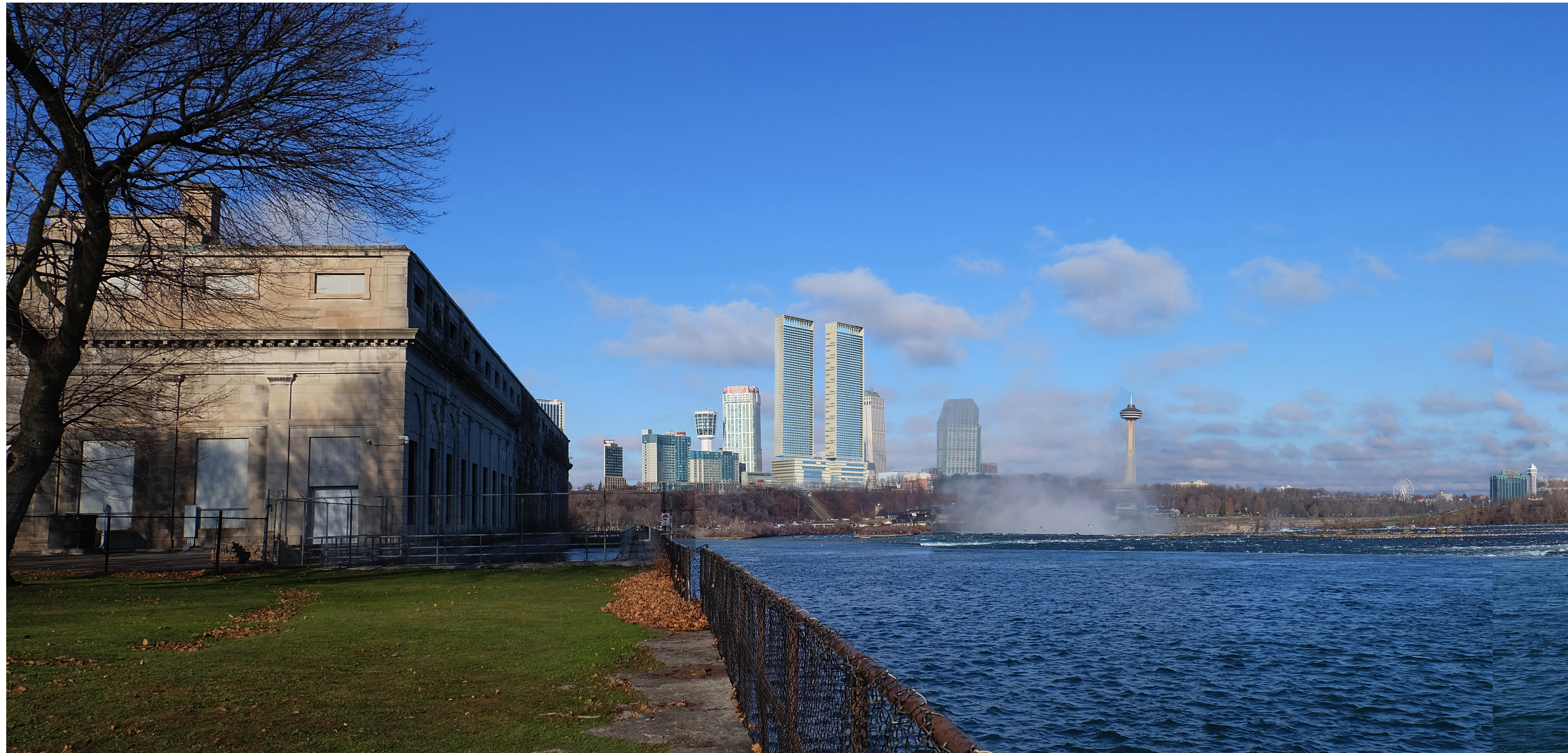
VIEW 01 - Looking North From the Old Power House
