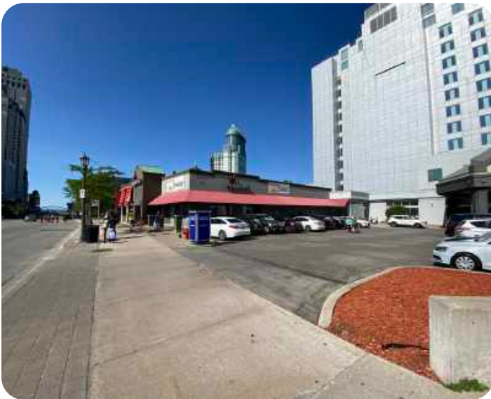
Looking north along the Hotel Site's Fallsview Boulevard frontage.
