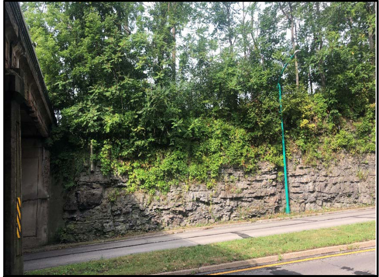
Figure 2: A section of the Slope with the Rock Cut
