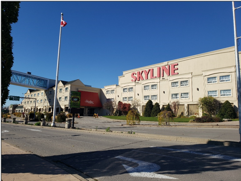
Figure 17 - Existing Three (3) storey hotel Immediately West of Subject Lands
