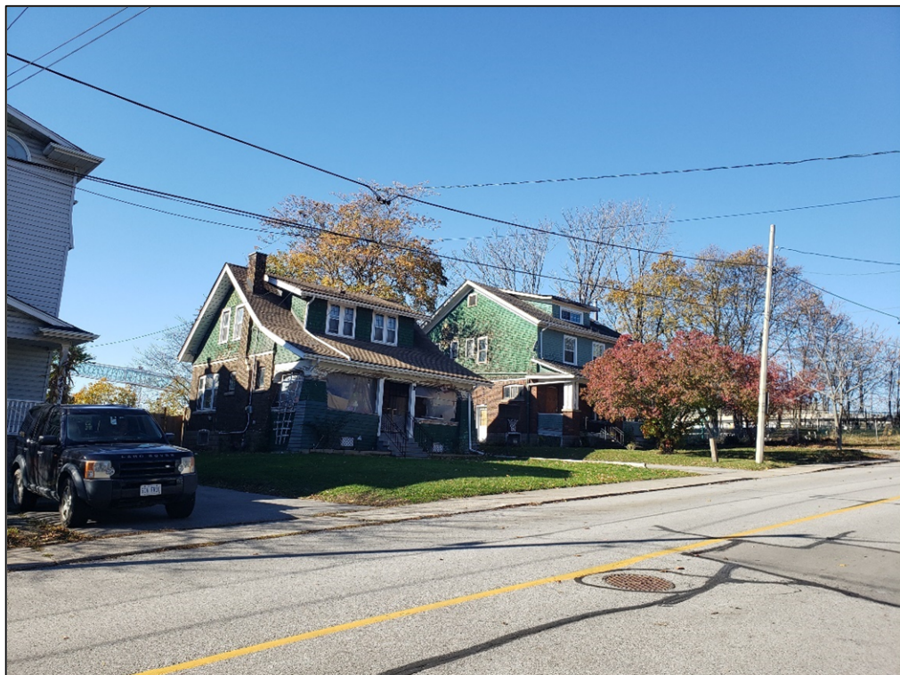
Figure 13 - Detached Dwellings on the West Side of Hiram Street
