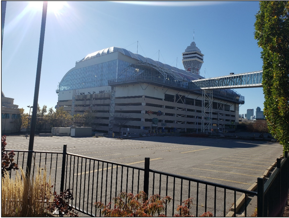
Figure 18 – Thirteen (13) Storey Casino Niagara Parking Garage, West ofo Subject Lands
